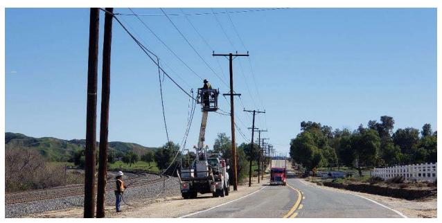
Photo 1 – SCE crew installing telecom fiber along San Timoteo Canyon Road for the El Casco Connection (February 19, 2019).
