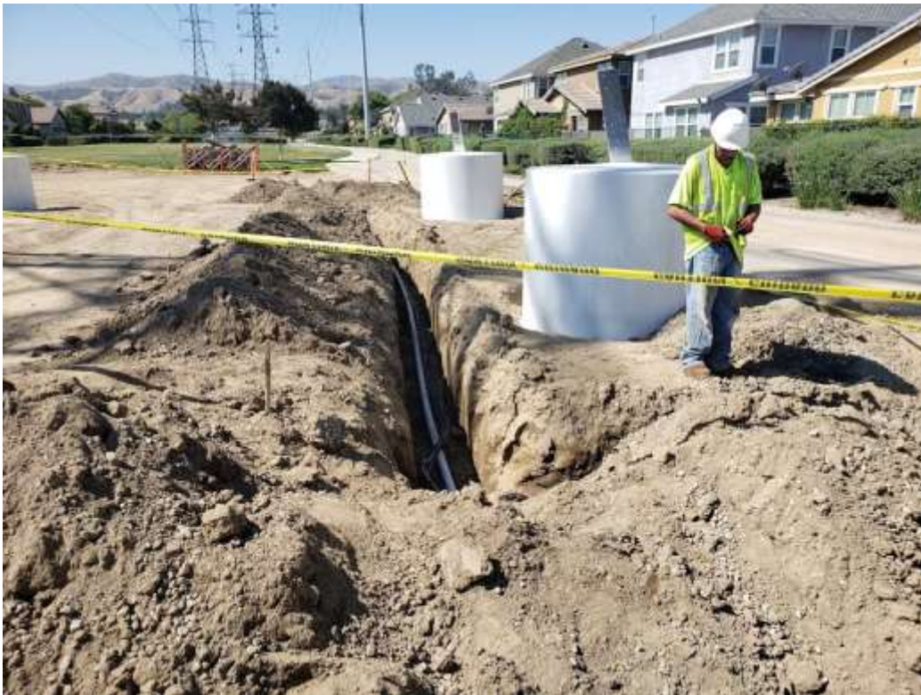
Photo 2 – irrigation repair on Segment 1 (June 12, 2019).
