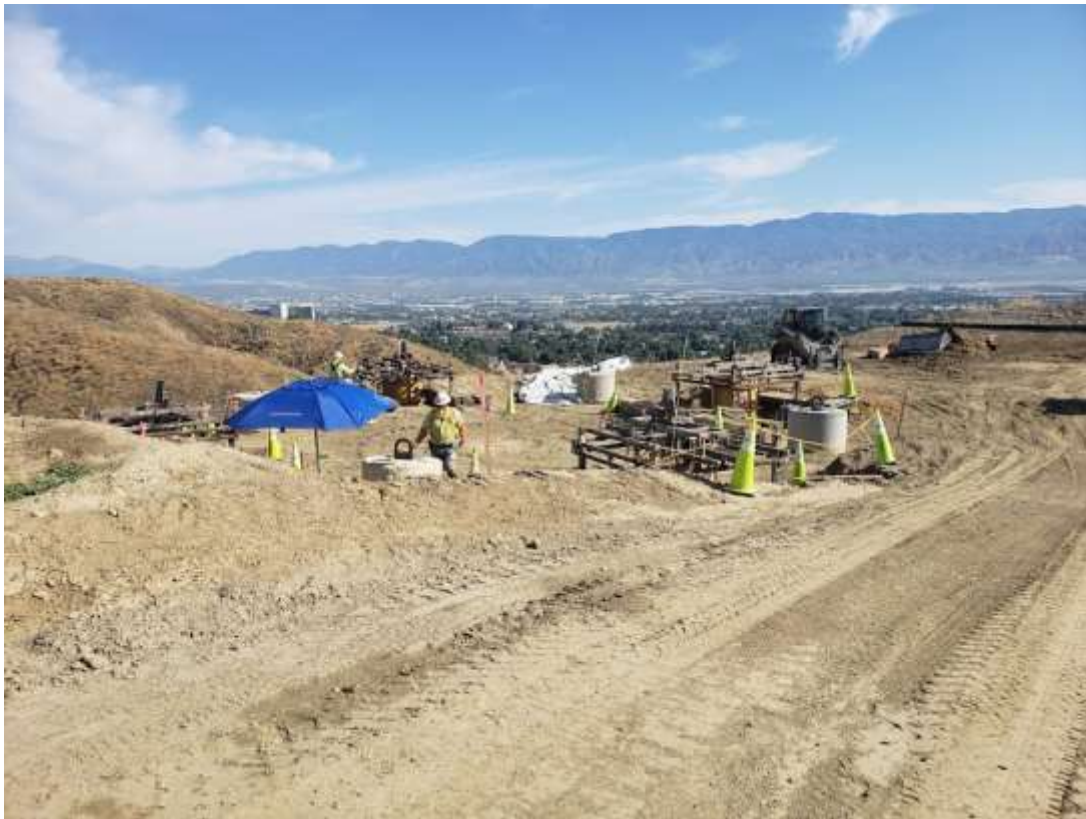
Photo 3 – Foundation activities on Segment 2 (June 11, 2019).
