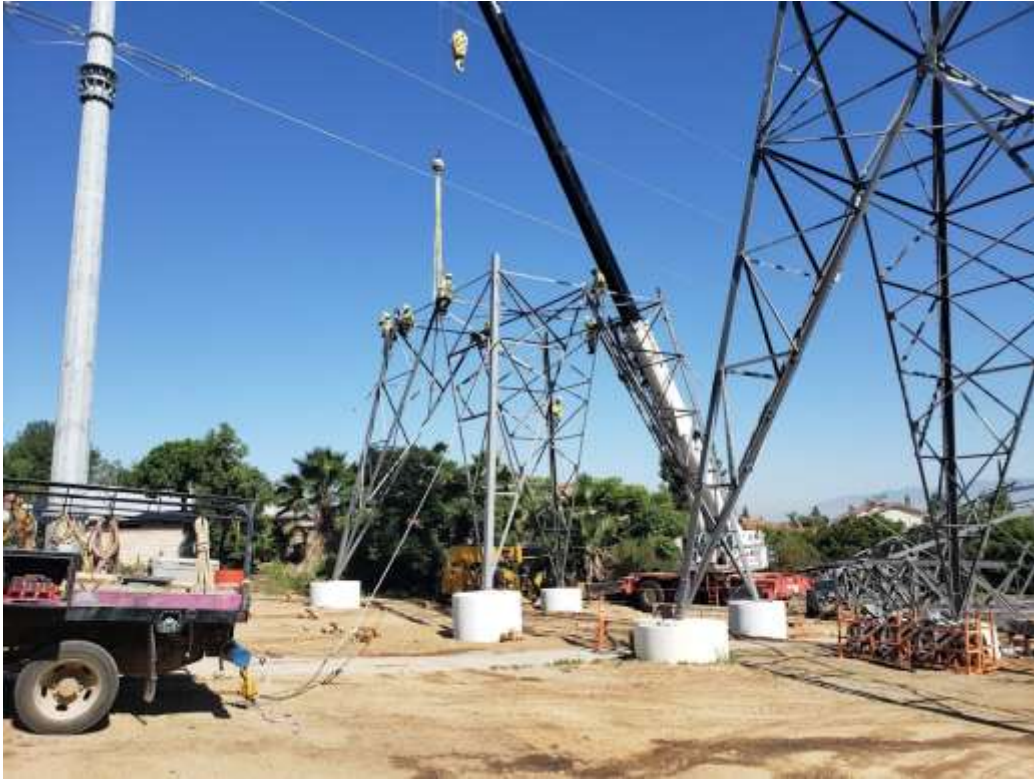
Photo 1 – Tower assembly activities on Segment 1 (June 12, 2019).
