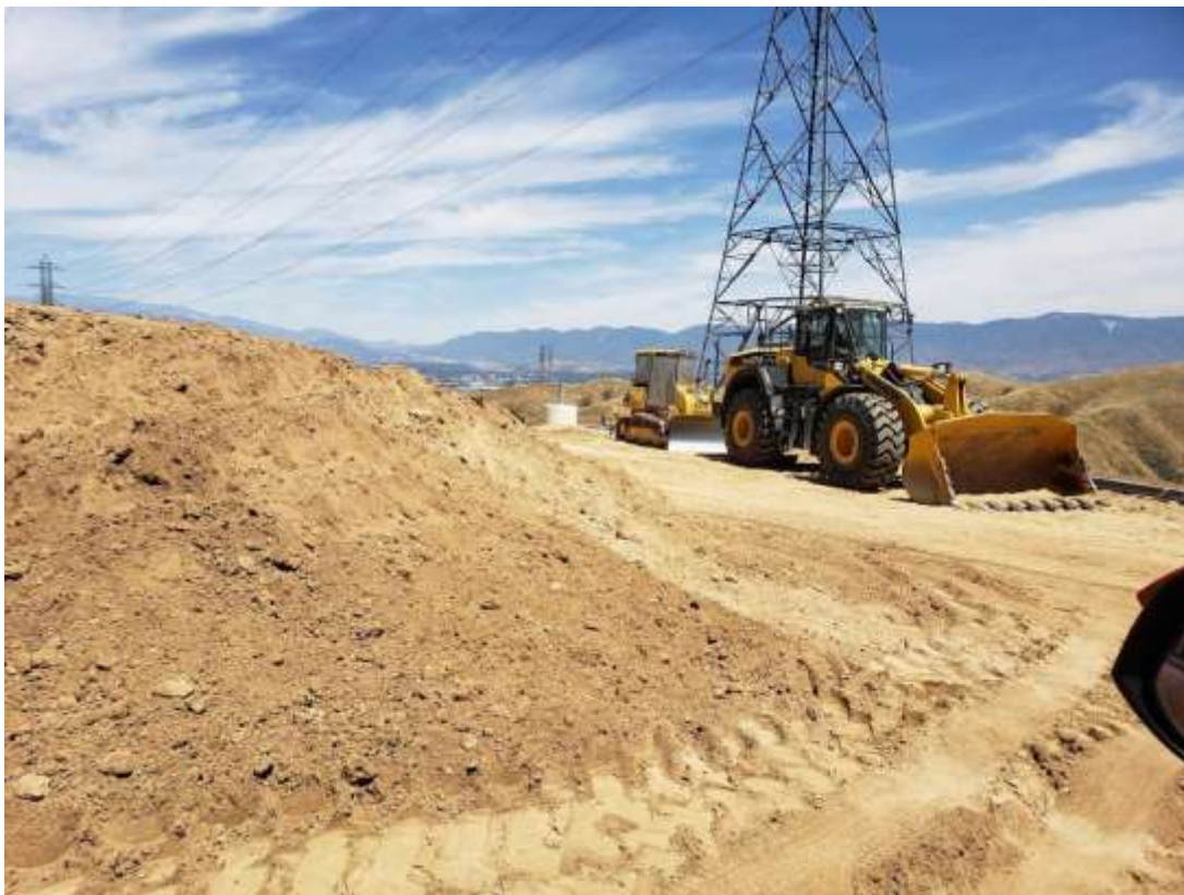
Photo 4 – Soil export preparation on Segment 3 (June 11, 2019).
