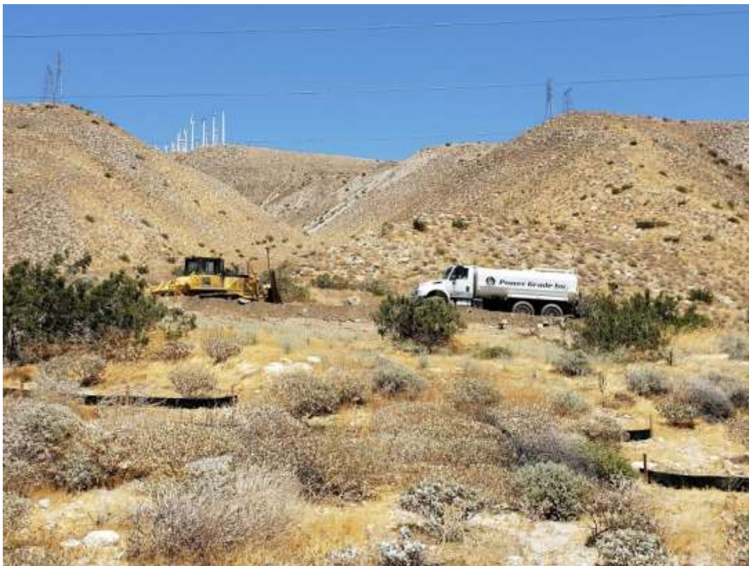
Photo 6 – Grading activities on Segment 6 (June 12, 2019).
