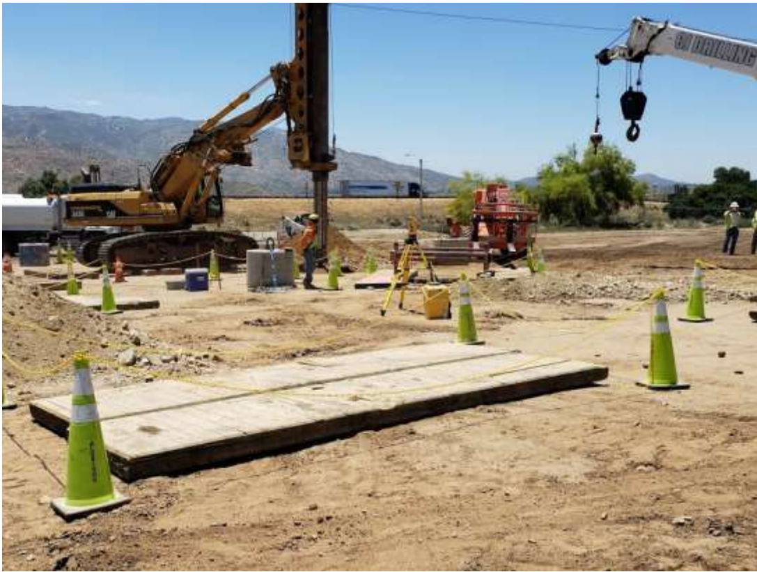
Photo 5 – Foundation activities on Segment 5 (June 12, 2019).
