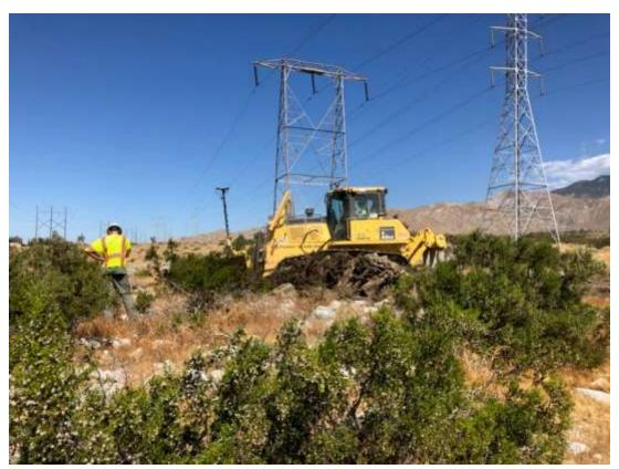
Photo 5 – Vegetation clearing and grading on Segment 6 (July 11, 2019).
