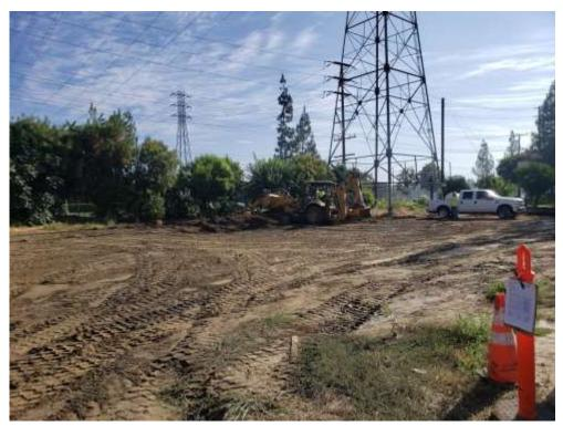
Photo 1 – Foundation wreck-out activities at Construction Area 1W18 on Segment 1 (July 30, 2019).
