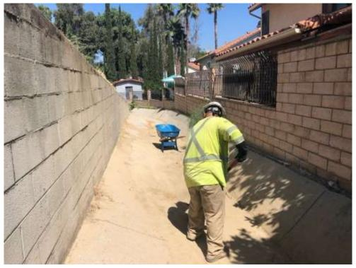
Photo 2 – Sediment removal from concrete v-ditch at TEWS #16 location near Construction Area 2X18 on Segment 2 (August 1, 2019).
