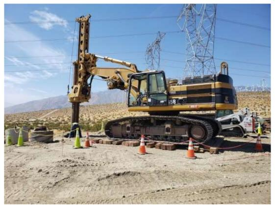
Photo 6 – Foundation drilling at Construction Area 6S19 on Segment 6 (July 30, 2019).
