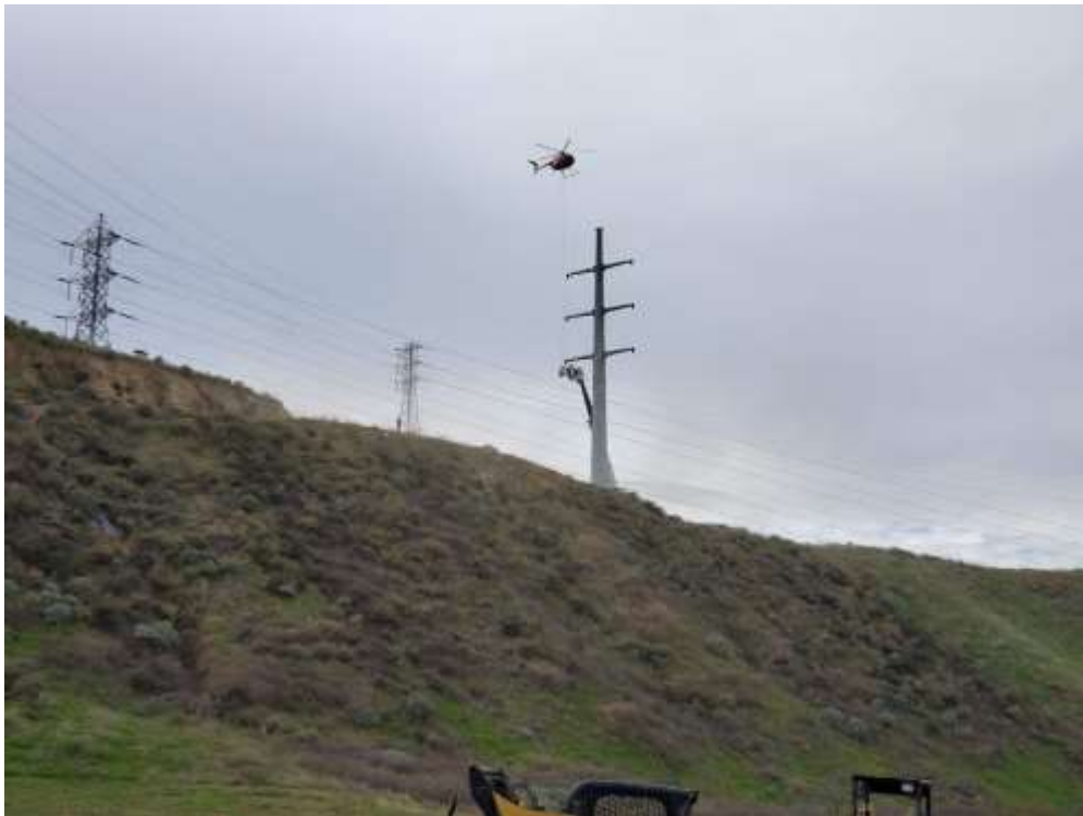
Photo 2 – Helicopter wire stringing activities at Construction Area 2N17, Segment 2 (January 20, 2020).
