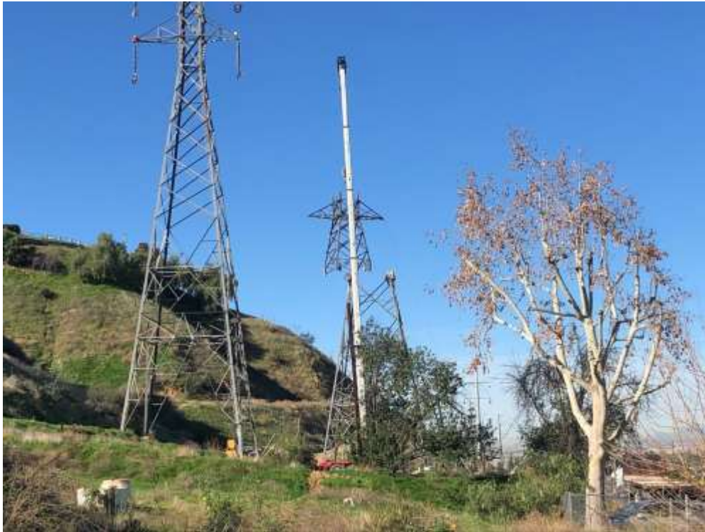
Photo 1 – Tower assembly at Construction Area 2N29, Segment 2 (January 24, 2020).
