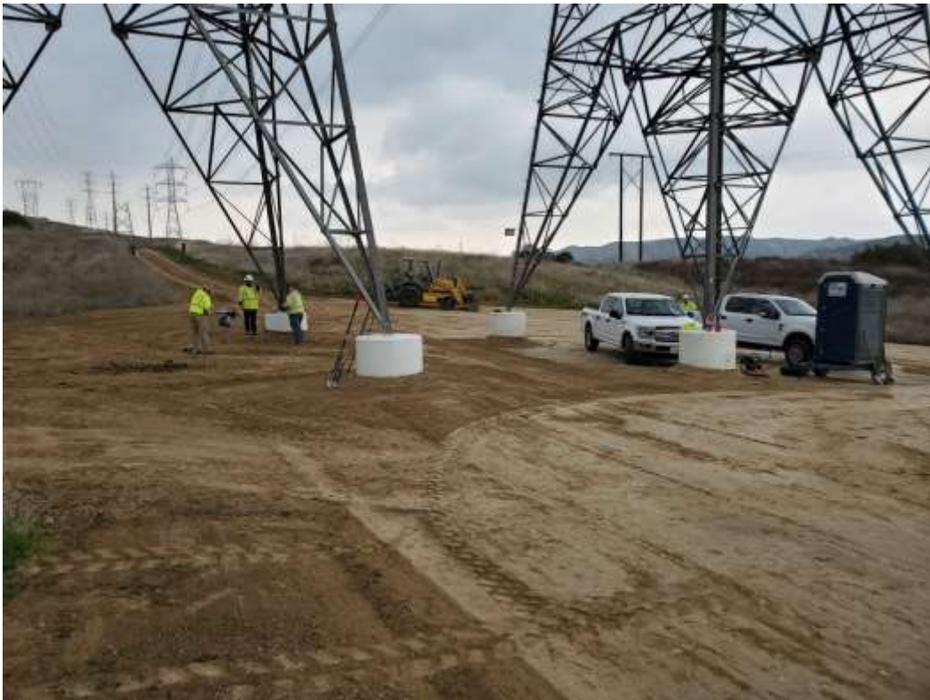
Photo 3 – Tower pad recontouring at Construction Area 3X14, Segment 3 (January 21, 2020).
