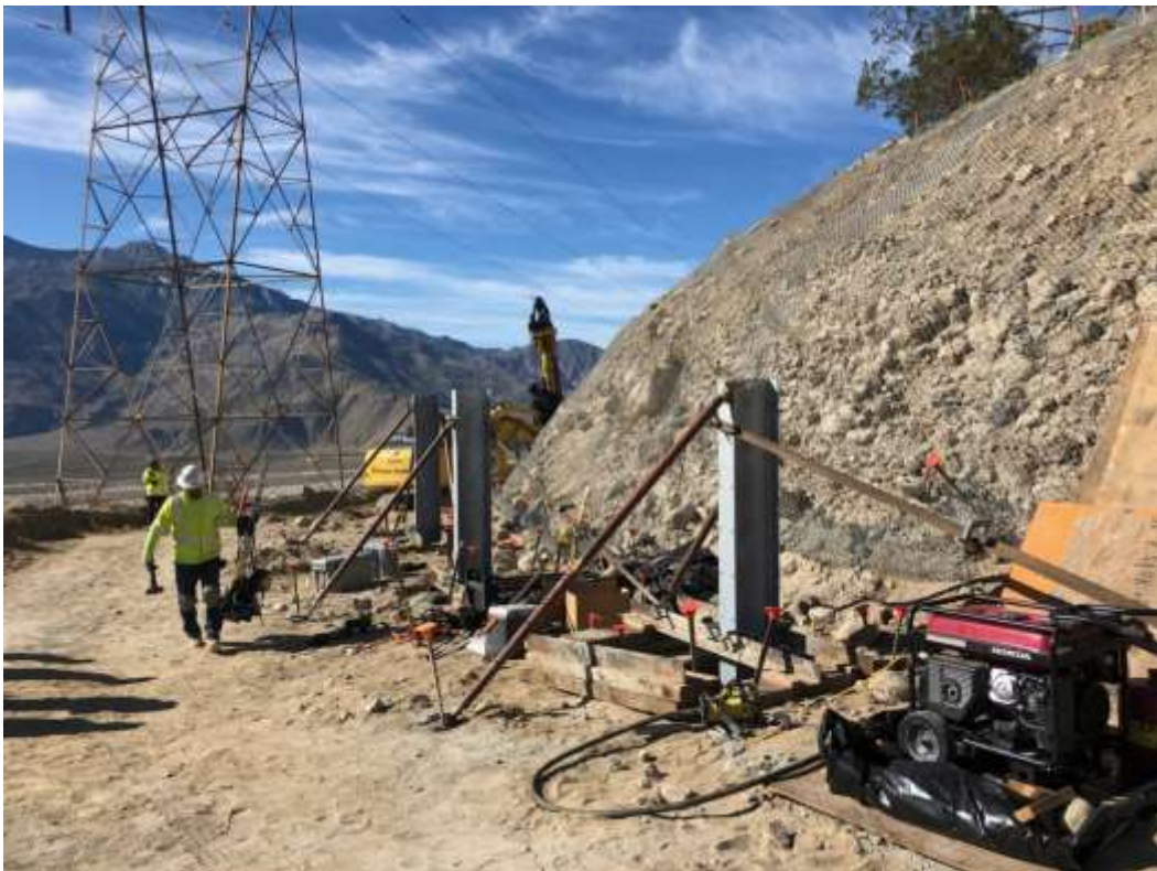
Photo 4 – Soldier pile wall construction at Construction Area 6N30, Segment 6 (January 23, 2020).
