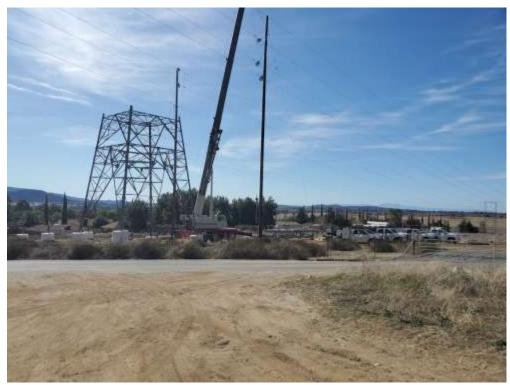
Photo 3 – Tower assembly at Construction Area 4X14, Segment 4. Note existing wire on shoofly towers (January 28, 2020).
