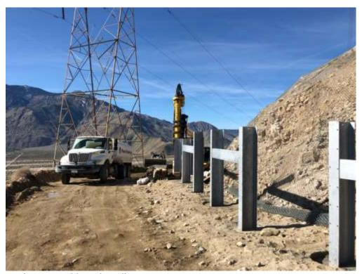
Photo 4 – Soldier pile wall construction at Construction Area 6N30, Segment 6 (January 31, 2020).
