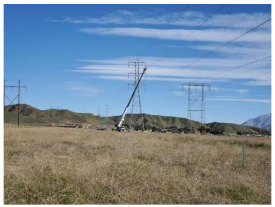
Photo 4 – Conductor wire transfer at Construction Area 4X18, Segment 4 (February 11, 2020).
