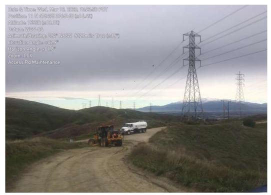
Photo 2 – Access road grading on Segment 2 between Construction Areas 2N01 and 2N18 (March 18, 2020) (Photo courtesy of SCE).
