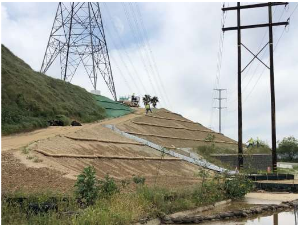
Photo 2 – Hydroseeding at Construction Area 2N32, Segment 2 (April 17, 2020).
