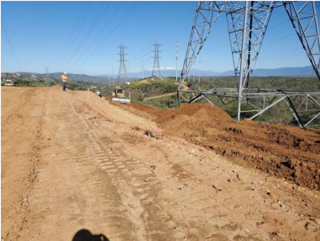
Photo 3 – Grading at Construction Area 4X55, Segment 4 (April 15, 2020).
