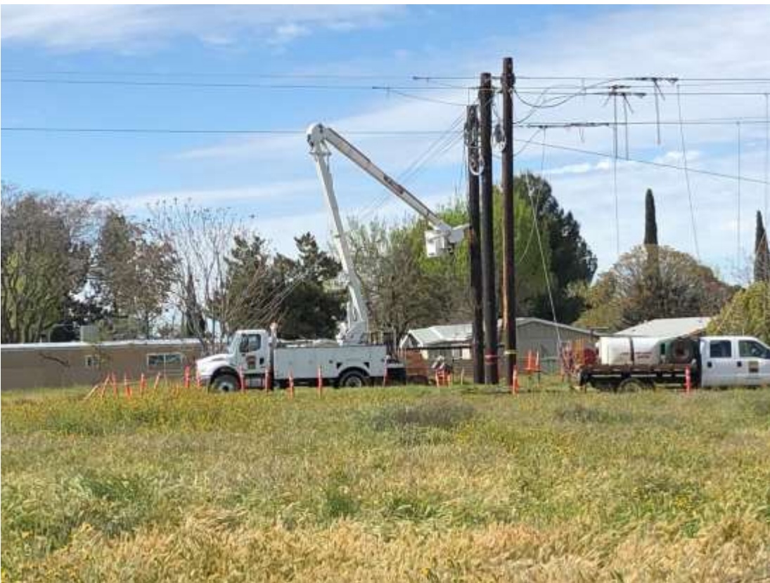
Photo 4 – Wire wreck-out activities at Construction Area WSS4X27-4X29, Segment 4 (April 17, 2020).
