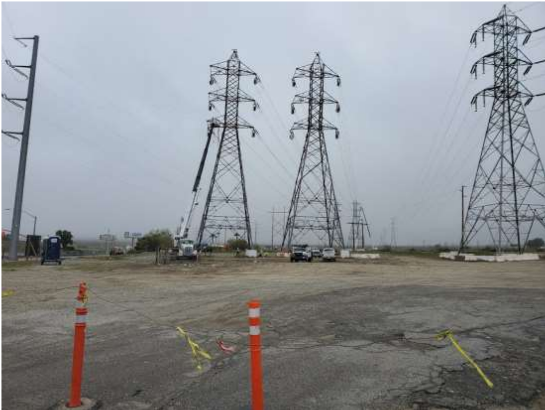
Photo 5 – Wire stringing activities at Construction Area 5X29, Segment 5 (April 13, 2020).
