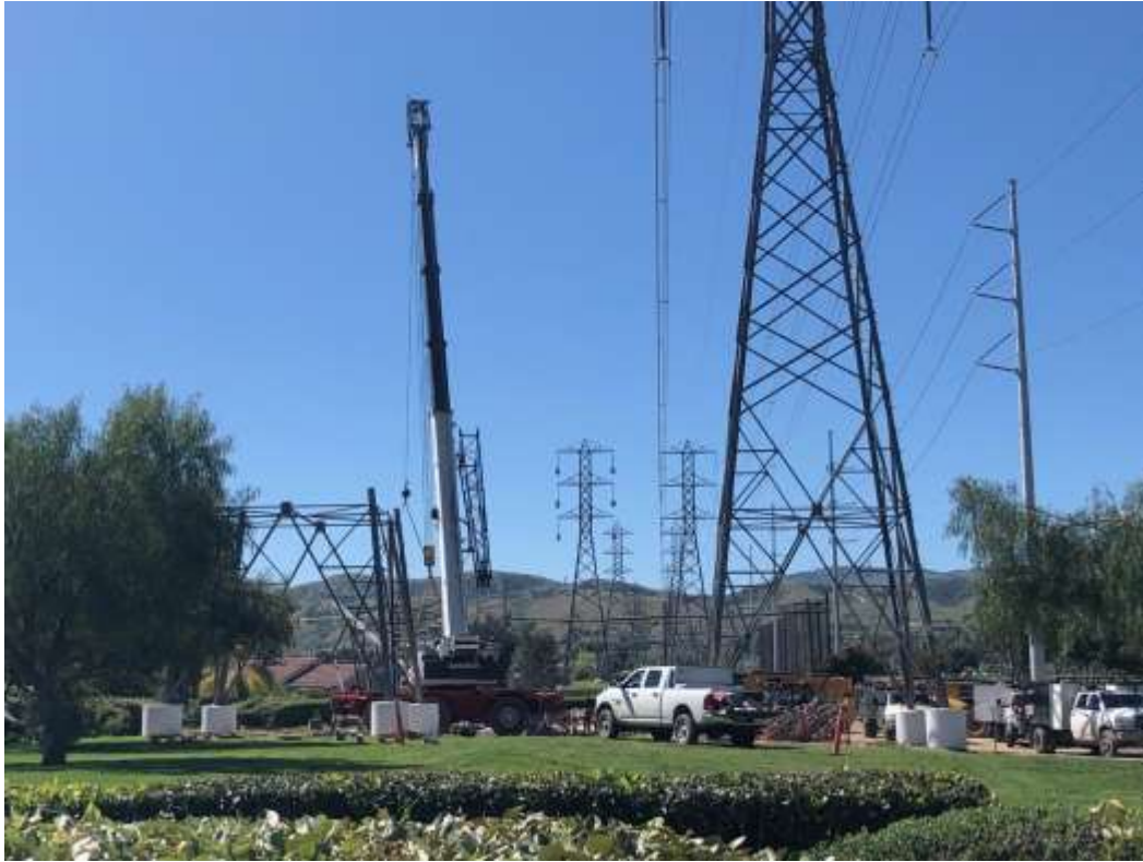
Photo 1 – Tower assembly at Construction Area 1X12, Segment 1 (April 16, 2020).
