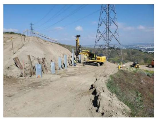
Photo 2 – Drilling piles at Construction Area 2N11, Segment 2 (April 21, 2020).
