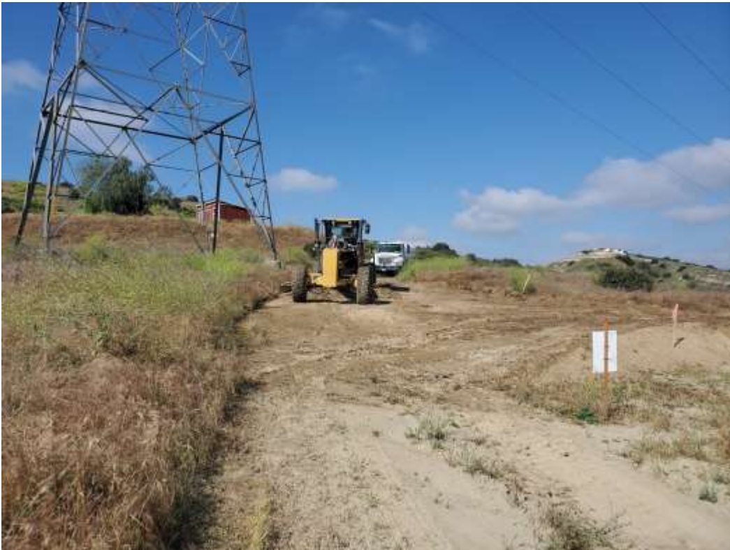
Photo 2 – Grading activities at Construction Area 3X23, Segment 3 (May 12, 2020).
