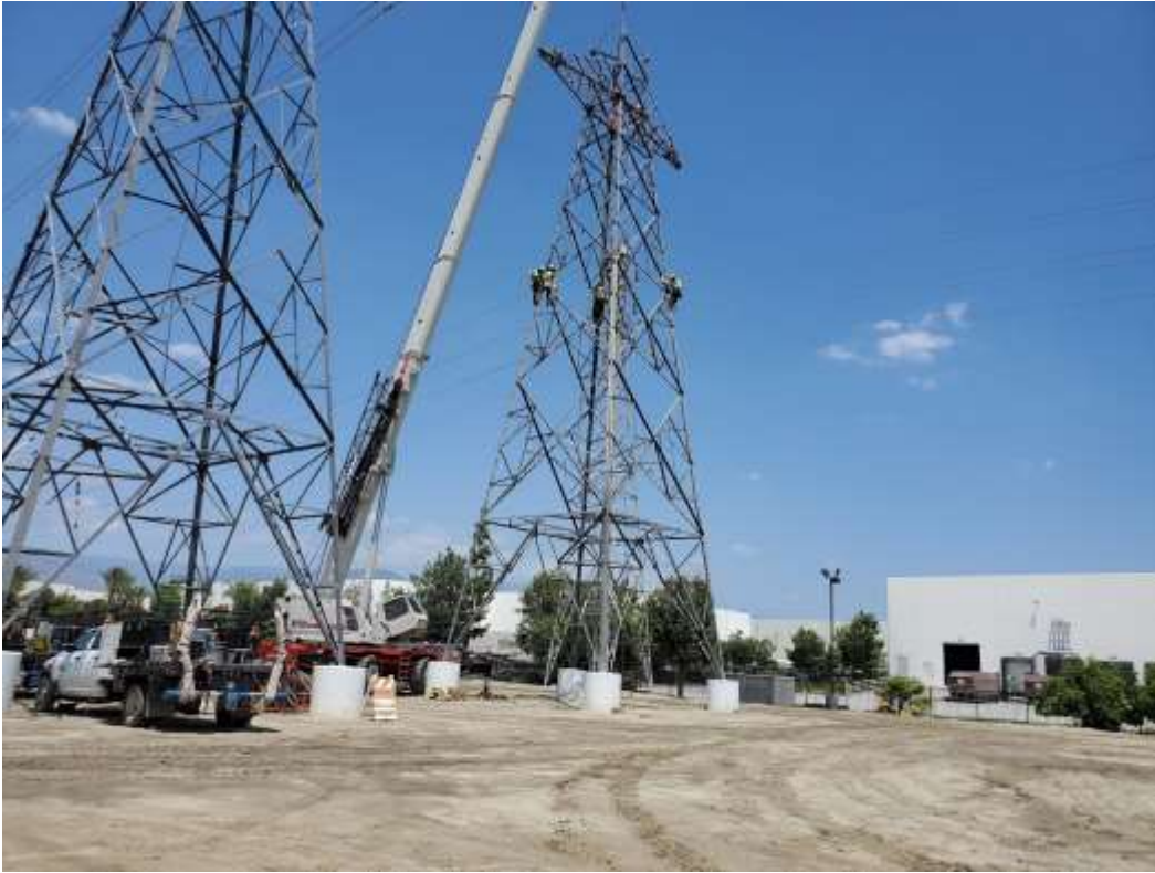
Photo 1 – Tower assembly at Construction Area 1X23, Segment 1 (May 13, 2020).
