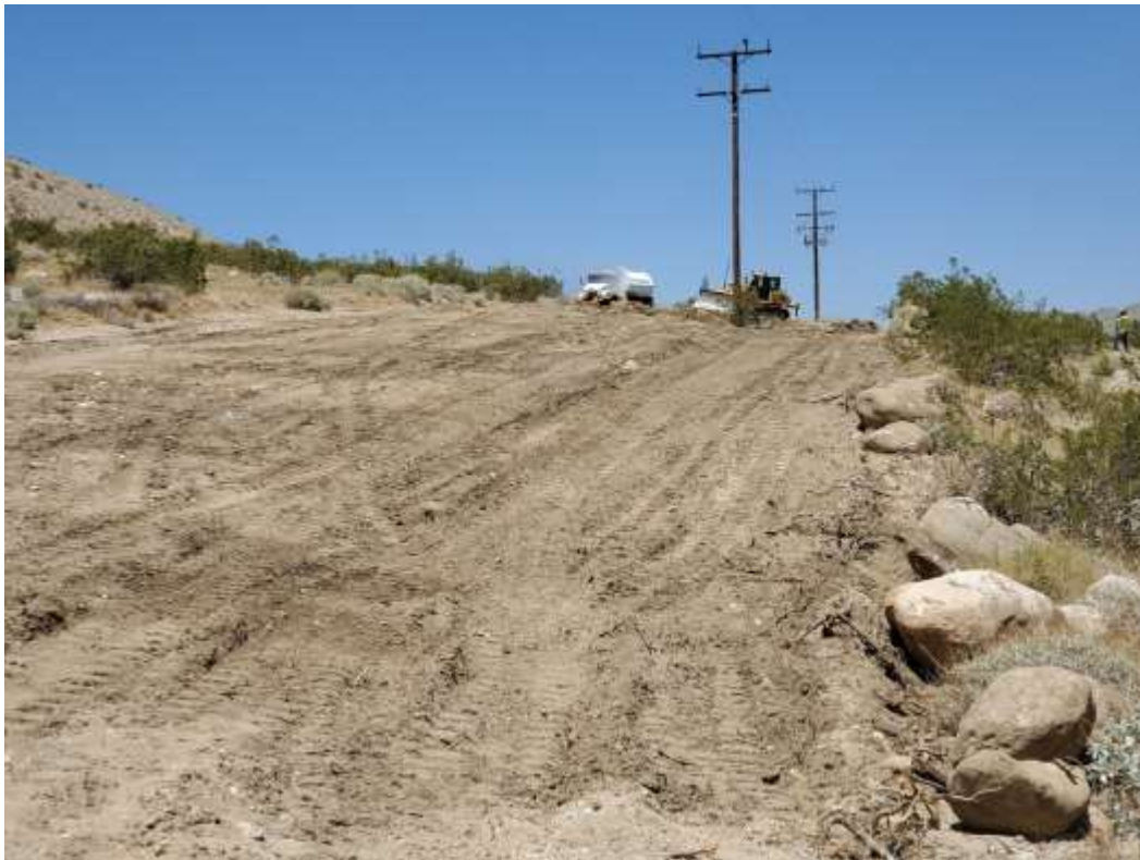
Photo 5 – Vegetation clearing and grading at Construction Area GS-6N27-6N28-3, Segment 6 (May 12, 2020).
