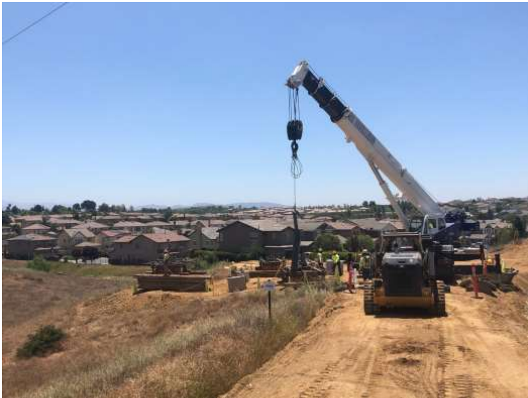
Photo 3 – Foundation activities at Construction Area 4X50, Segment 4 (May 15, 2020).
