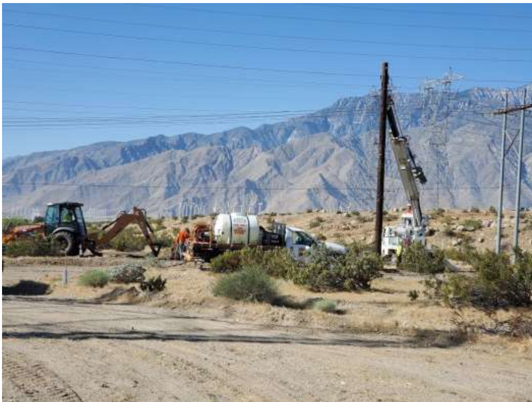
Photo 6 – Snub removal activities at Construction Area 6X11, Segment 6 (May 11, 2020).
