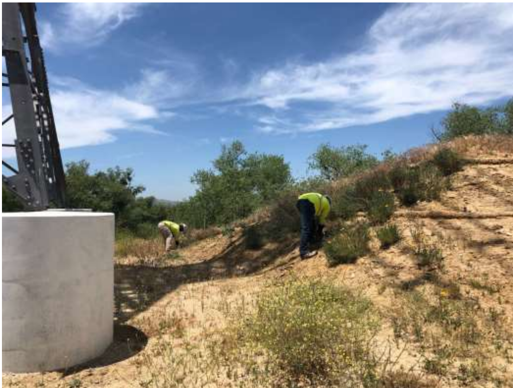
Photo 4 – Hand weeding at Construction Area 4N62 Segment 4 (May 14, 2020).
