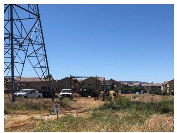
Photo 4 – Foundation wreck-out activities at Construction Area 4X26, Segment 4 (May 21, 2020).
