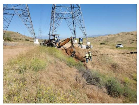
Photo 2 – MAC drain installation at Construction Area 3X59, Segment 3 (May 20, 2020).
