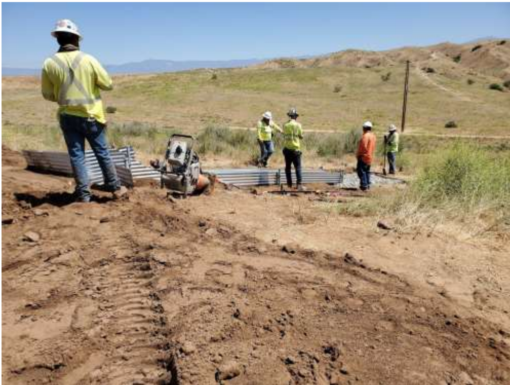
Photo 2 – MAC drain installation at Construction Area 3X61, Segment 3 (May 27, 2020).
