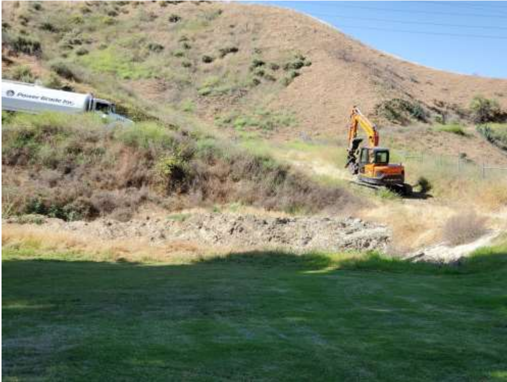
Photo 1 – Erosion repair at Construction Area 2N18, Segment 2 (May 27, 2020).
