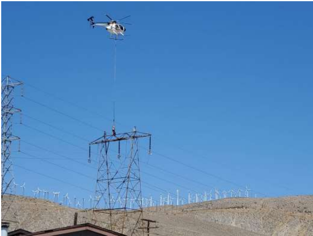
Photo 5 – Helicopter wire wreck-out activities at Construction Area 6N40, Segment 6 (May 26, 2020).
