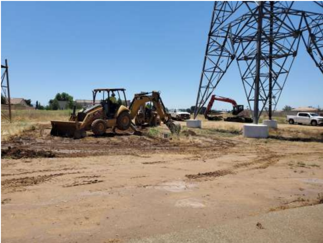
Photo 3 – Foundation wreck-out activities at Construction Area 4X30, Segment 4 (May 27, 2020).
