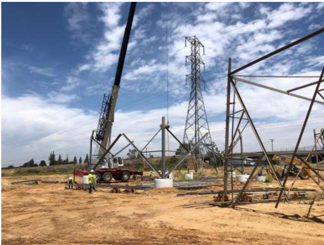
Photo 4 – Tower assembly at Construction Area 4X45, Segment 4 (May 29, 2020).
