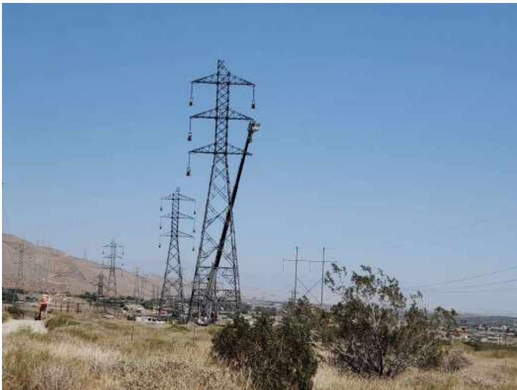
Photo 6 – Wire stringing activities at Construction Area 6X47, Segment 6 (May 27, 2020).
