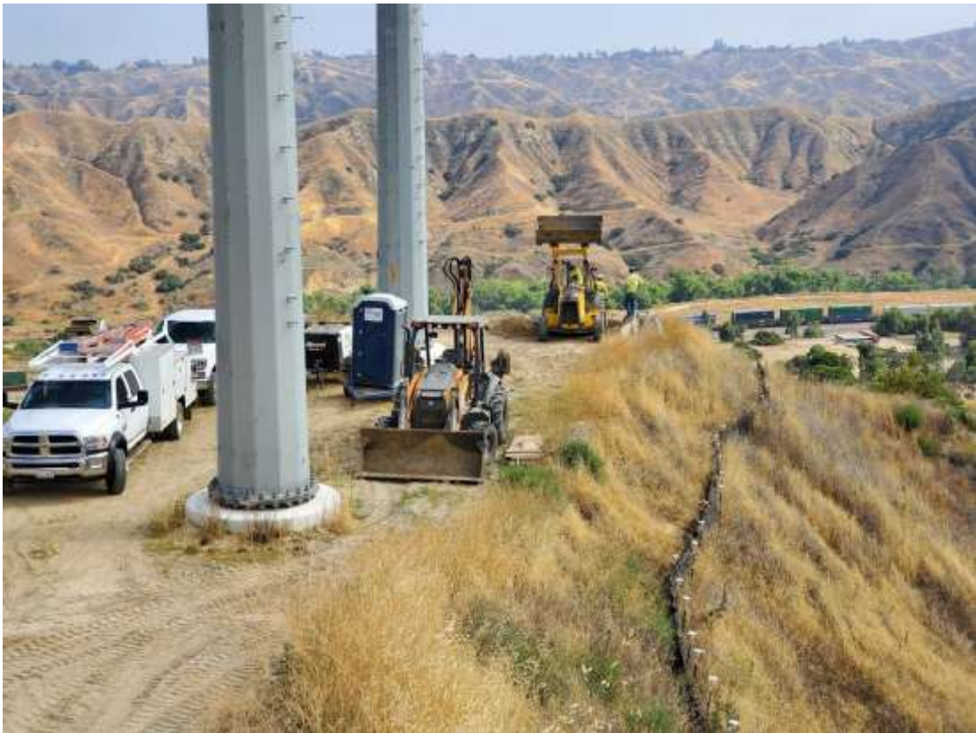
Photo 3 – MAC drain installation at Construction Area 3X35, Segment 3 (June 16, 2020).
