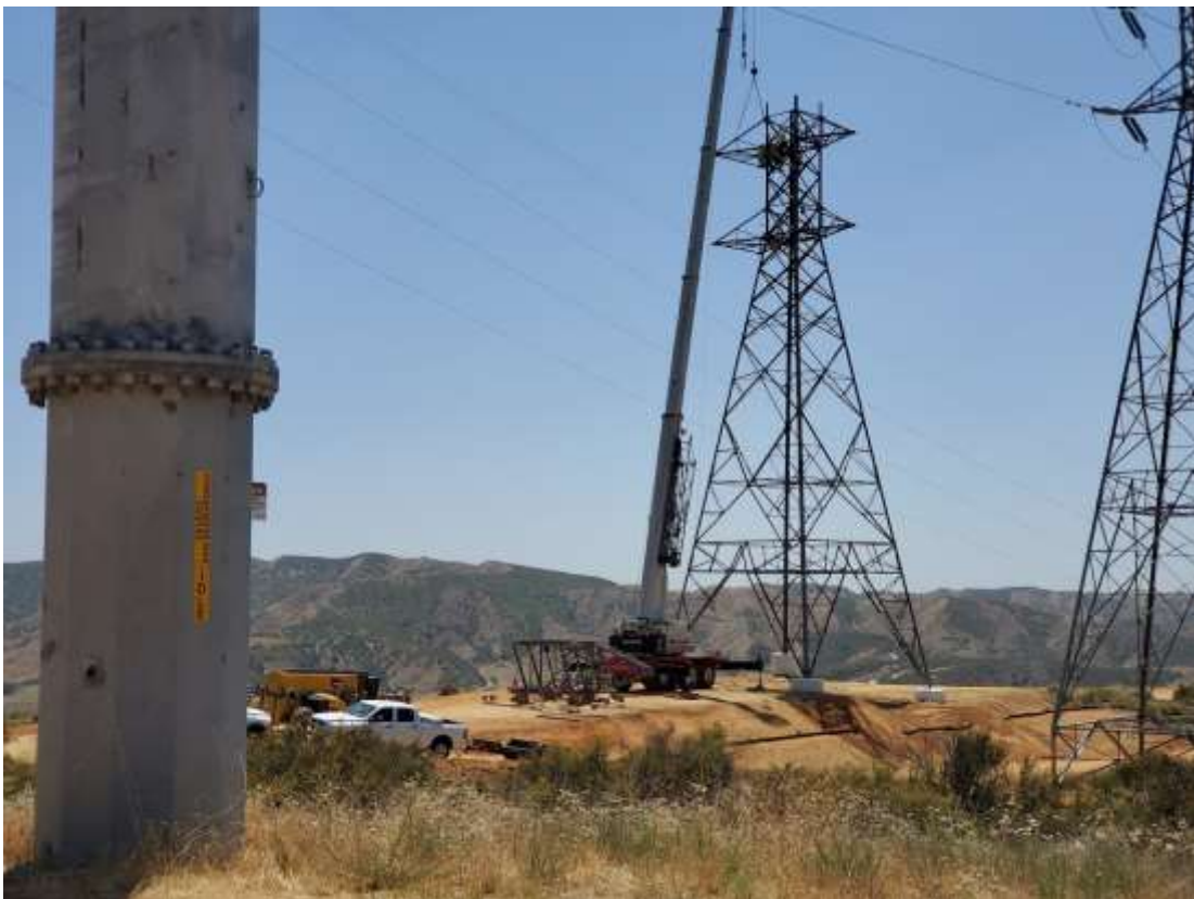
Photo 4 – Tower assembly at Construction Area 4X56, Segment 4 (June 15, 2020).
