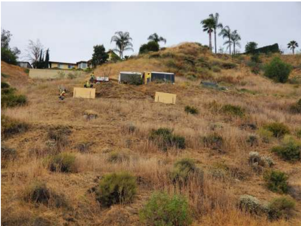
Photo 2 – Foundation removal at Construction Area 2N32, Segment 2 (June 16, 2020).
