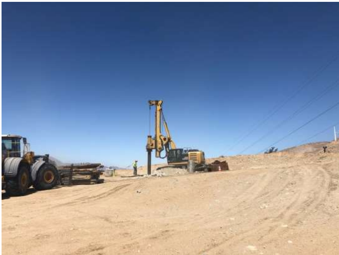
Photo 6 – Foundation activities at Construction Area 6N28, Segment 6 (June 18, 2020).
