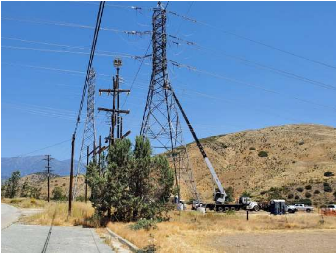
Photo 5 – Wire stringing activities at Construction Area 4X01, Segment 4 (June 15, 2020).
