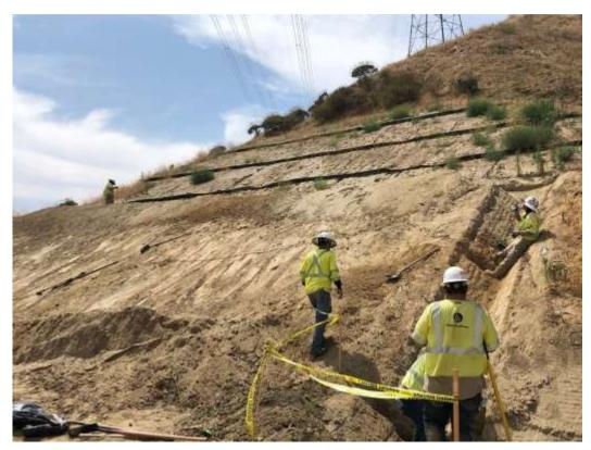
Photo 2 – V-ditch preparation activities at Construction Area 2N18, Segment 2 (June 25, 2020).
