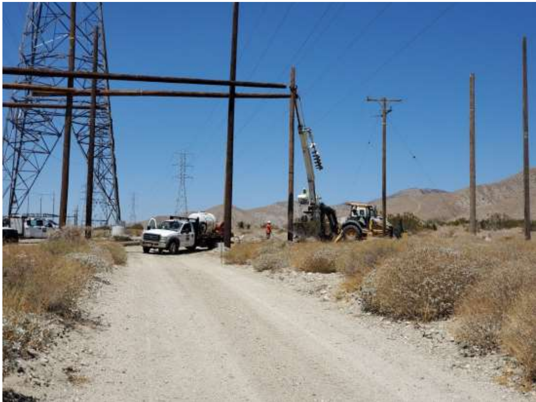
Photo 6 – Guard pole installation at Construction Area 6X46, Segment 6 (July 22, 2020).
