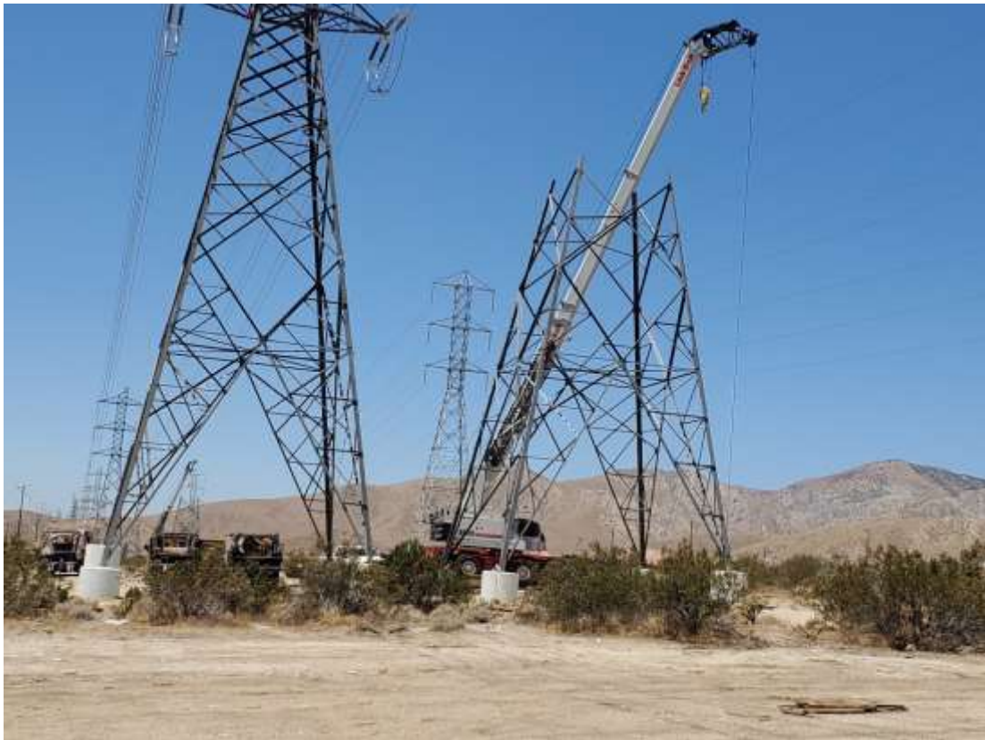
Photo 5 – Tower assembly at Construction Area 5X01, Segment 5 (July 22, 2020).
