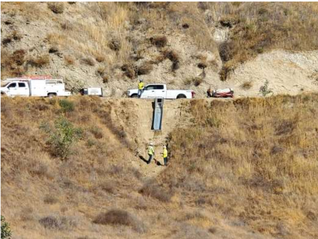
Photo 2 – MAC drain installation at Construction Area 3X19, Segment 3 (July 21, 2020).
