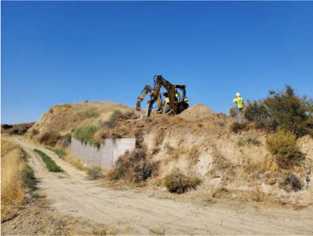
Photo 1 – Foundation removal activities at Construction Area 3X35, Segment 3 (July 22, 2020).
