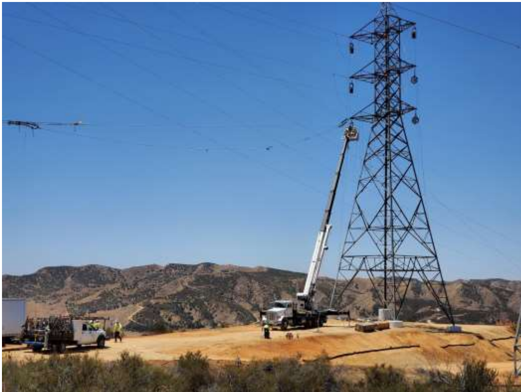
Photo 3 – Wire stringing activities at Construction Area 4X56, Segment 4 (July 20, 2020).
