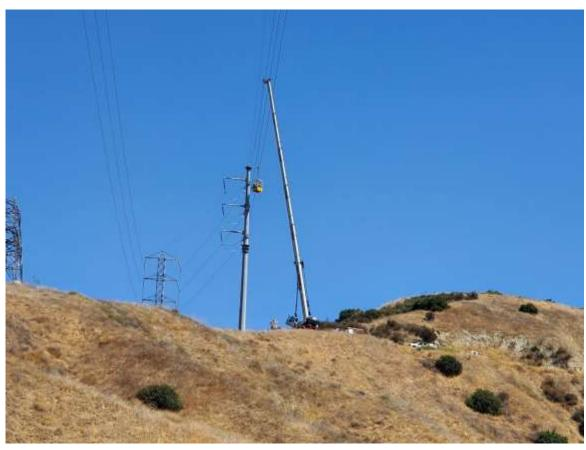
Photo 3 – Bridle conductor activities at Construction Area SF305, Segment 3 (August 10, 2020).
