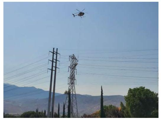
Photo 4 – Wire wreck-out activities at Construction Area 4X03, Segment 4 (September 2, 2020).
