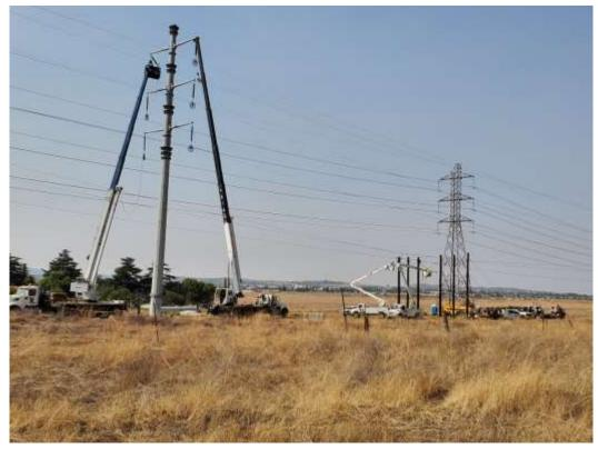
Photo 3 – Wire wreck-out activities at Construction Area WSS-4X15-4X16, Segment 4 (September 14, 2020).
