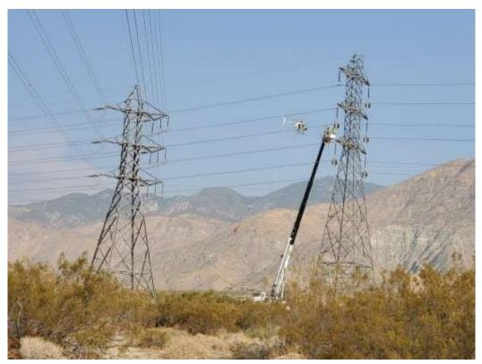
Photo 6 – Wire stringing activities and helicopter operations at Construction Area 6N42, Segment 6 (September 14, 2020).
