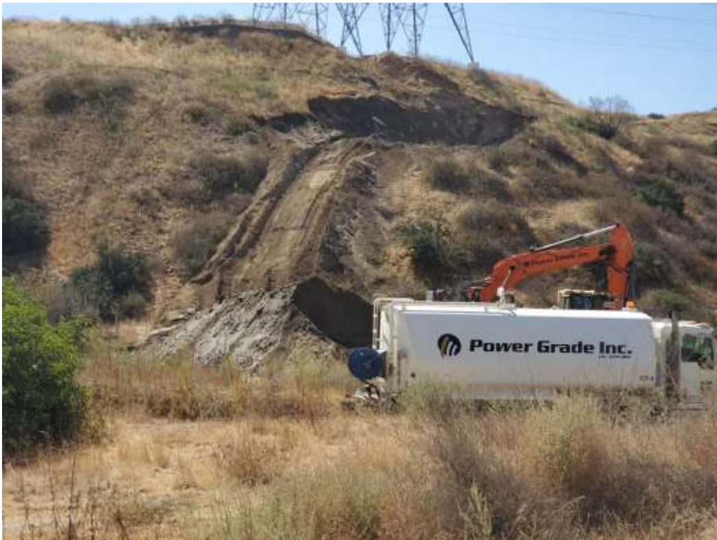
Photo 2 – Erosion repair activities at Construction Area 3X64, Segment 3 (September 29, 2020).
