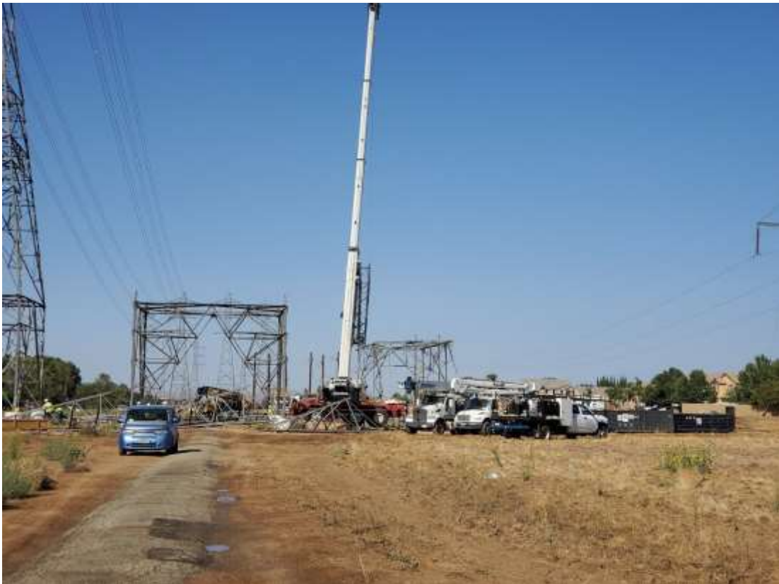
Photo 4 – Tower assembly at Construction Area 4X27, Segment 4 (September 28, 2020).
