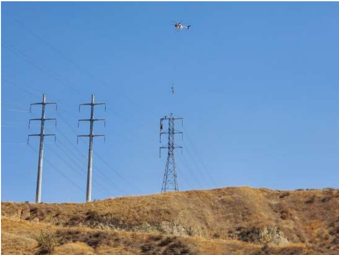
Photo 3 – Wire wreck-out activities at Construction Area 3X46, Segment 3 (September 30, 2020).
