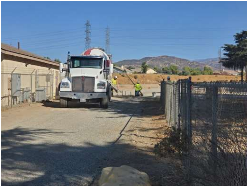
Photo 6 – Conduit installation activities at Construction Area TWA-4S35X-1, Segment 4 (September 30, 2020).
