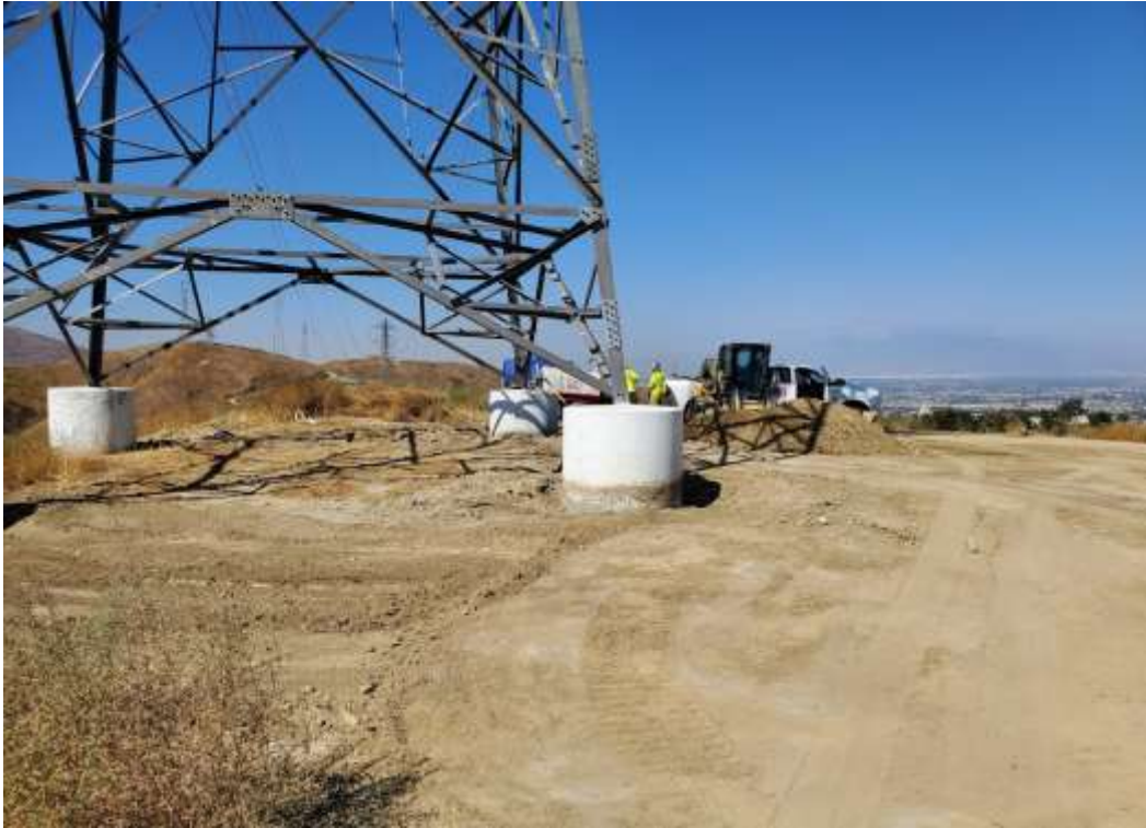
Photo 1 – Site restoration activities at Construction Area 2N08, Segment 2 (September 30, 2020).
