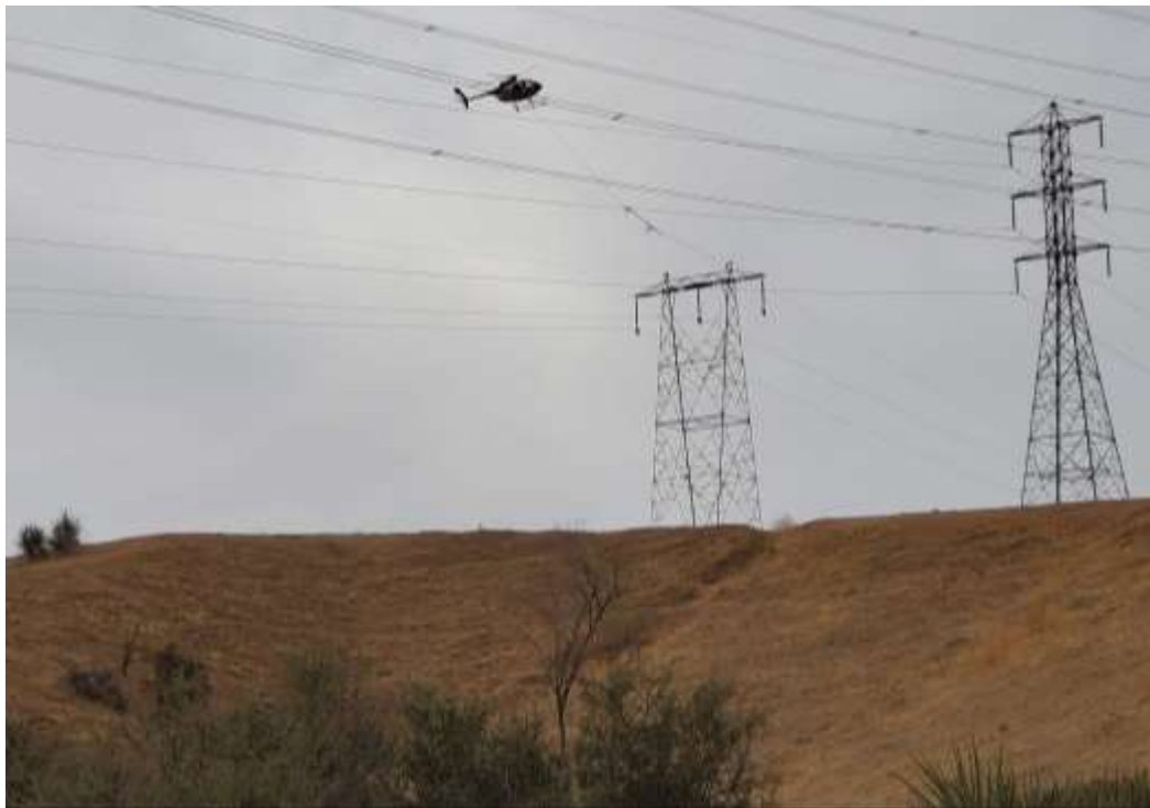
Photo 2 – Helicopter wire wreck-out activities at Construction Area 3X59, Segment 3 (December 7, 2020).
