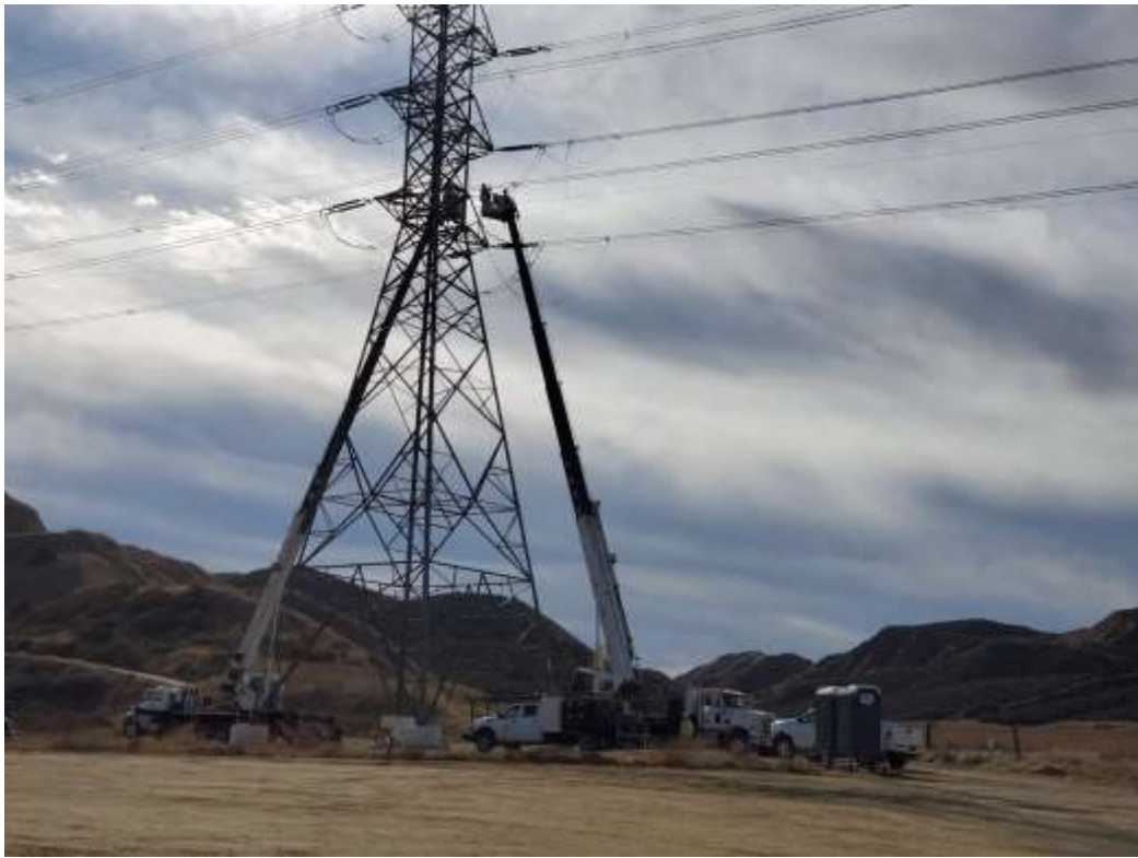
Photo 3 – Wire stringing activities at Construction Area 3X06, Segment 3 (December 8, 2020).
