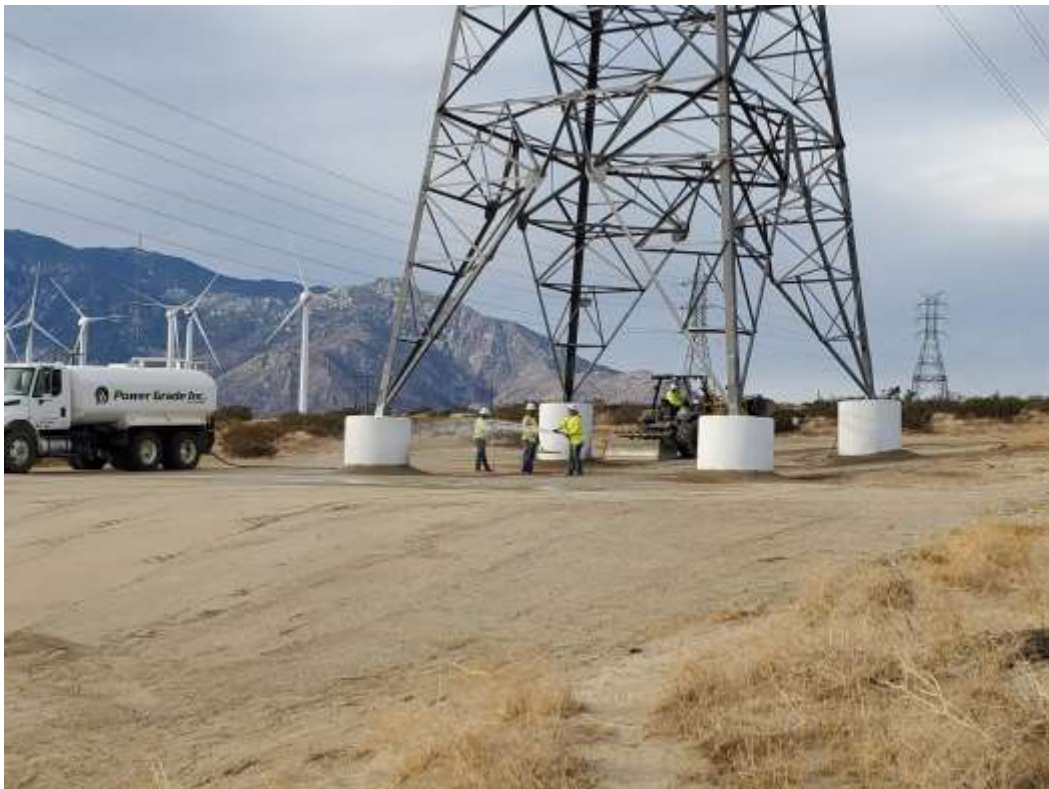
Photo 6 – Site restoration activities at Construction Area 6N25, Segment 6 (December 9, 2020).
