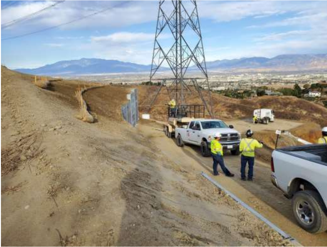
Photo 1 – Hydroseed application at Construction Area 2N11, Segment 2 (December 8, 2020).
