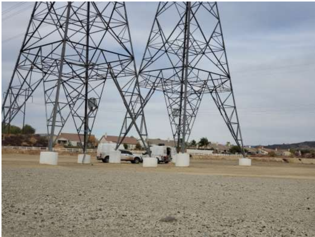
Photo 4 – Testing and splicing fiber at Construction Area 4X35, Segment 4 (December 9, 2020).
