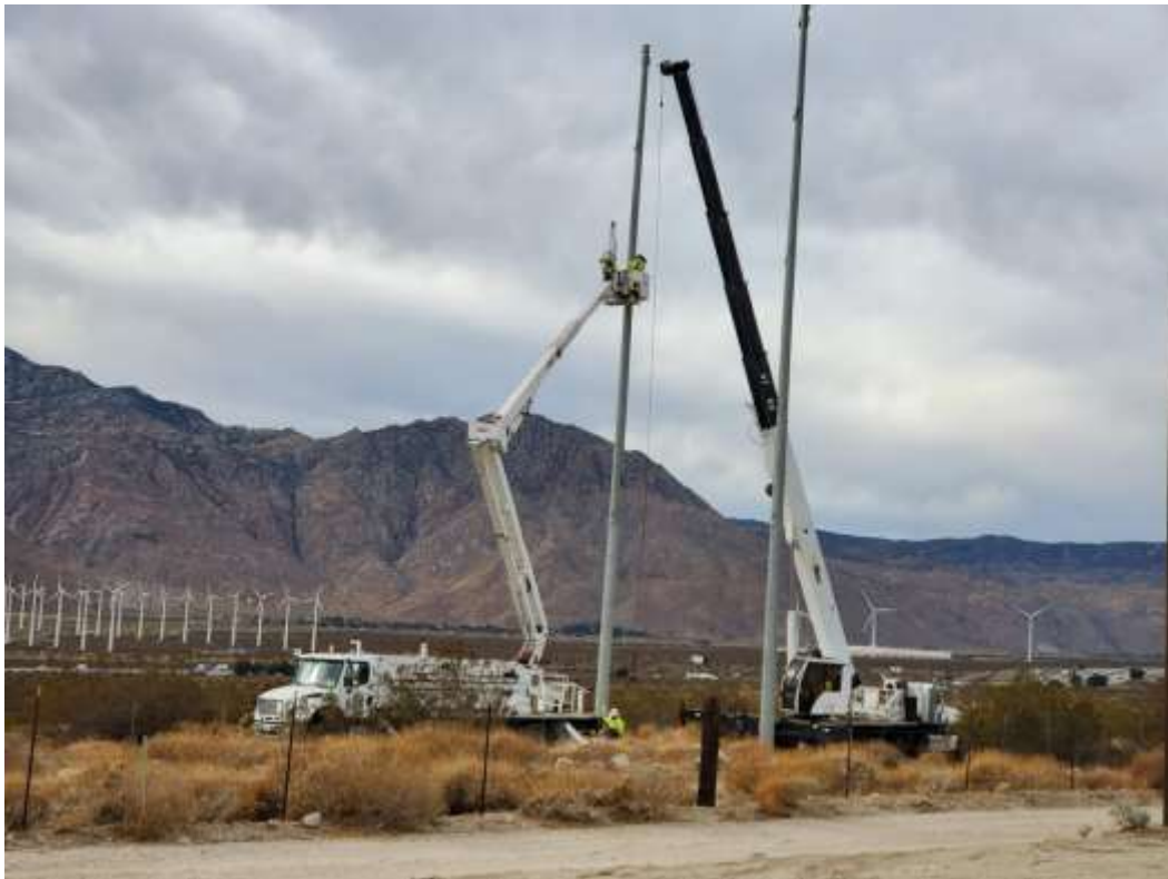
Photo 5 – H-frame wreck-out at Construction Area 5X01, Segment 5 (December 7, 2020).
