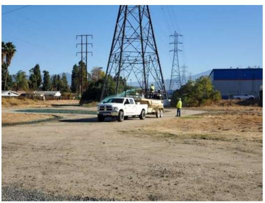
Photo 2 – Hydroseed application at Construction Area 2N35, Segment 2 (December 15, 2020).
