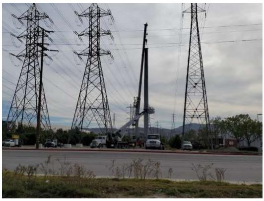
Photo 2 – Shoofly tower wreck-out at Construction Area 1X25, Segment 1 (January 13, 2021).
