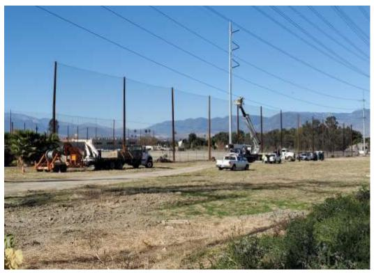
Photo 1 – Wire wreck-out activities at Construction Areas 1X10 through 1X11, Segment 1 (January 14, 2021).
