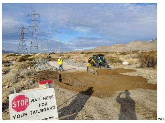
Photo 6 – Backfilling activities at wet crossing on access road to 6X42, Segment 6 (January 27, 2021).
