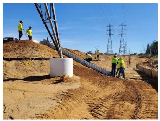
Photo 3 – MAC drain installation at Construction Area 4X47, Segment 4 (February 8, 2021).
