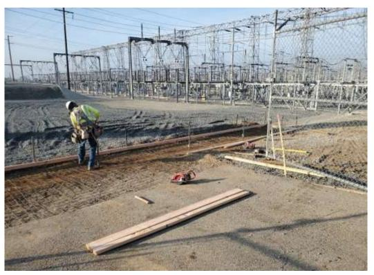
Photo 1 – Concrete form installation for V-ditch at Construction Area 2N39, Segment 2 (February 11, 2021).
