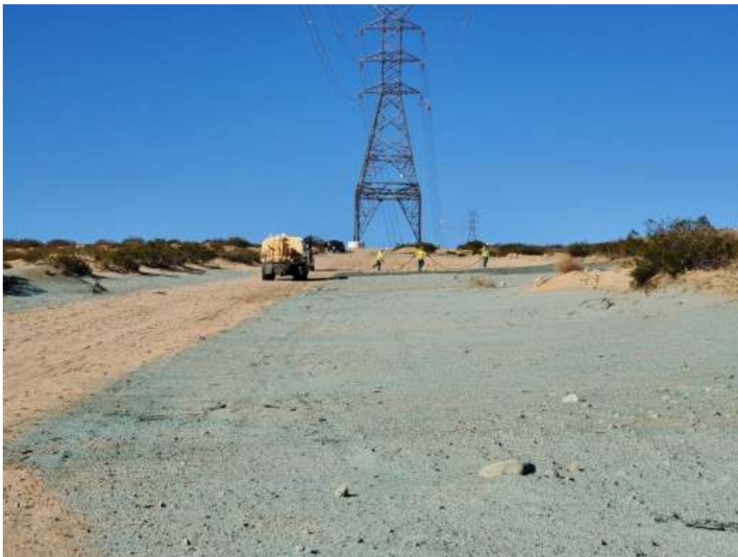
Photo 6 – Hydroseed application at Construction Area WSS-6-6S26-2-MPR-29, Segment 6 (February 24, 2021).
