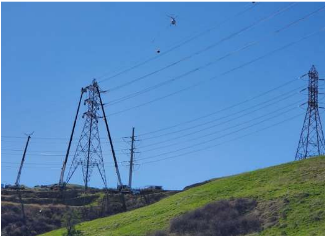
Photo 2 – Helicopter wire stringing activities at Construction Area 2N02, Segment 2 (February 22, 2021).
