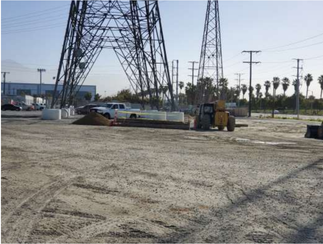
Photo 1 – Shoofly foundation wreck-out at Construction 1X26 (SF130), Segment 1 (February 25, 2021).
