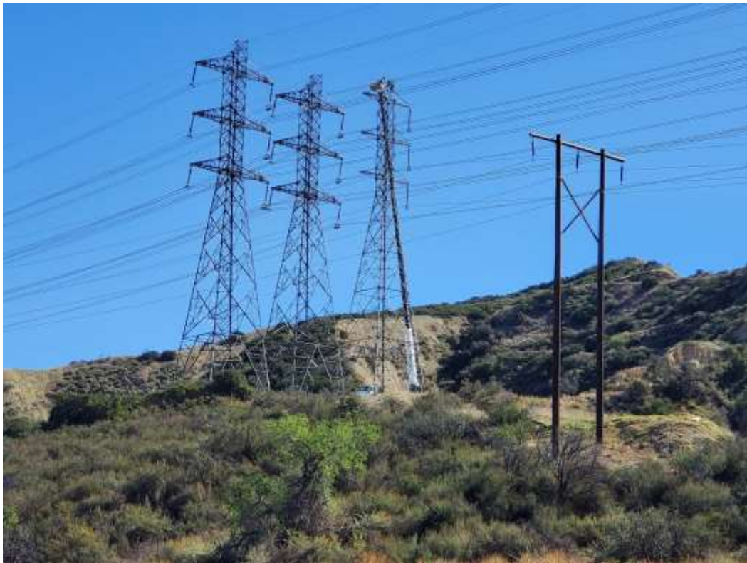
Photo 3 – Wire wreck-out activities at Construction Area 3X21, Segment 3 (February 22, 2021).
