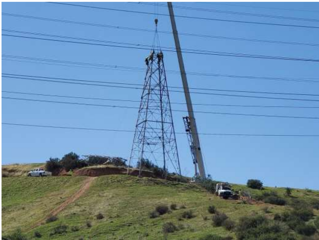
Photo 4 – Tower wreck-out at Construction Area M38-T4, Segment 3 (February 24, 2021).
