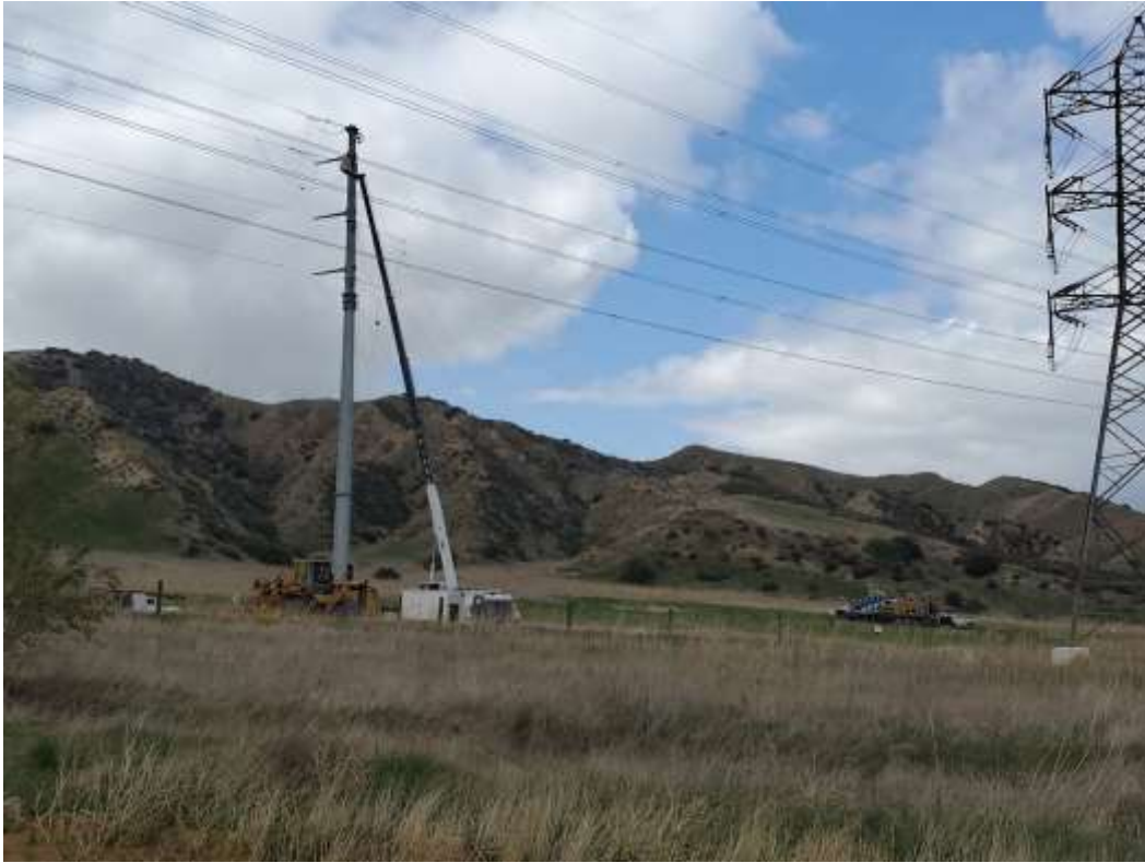
Photo 1 – Wire wreck-out activities at Construction Area 3X07, Segment 3 (March 8, 2021).
