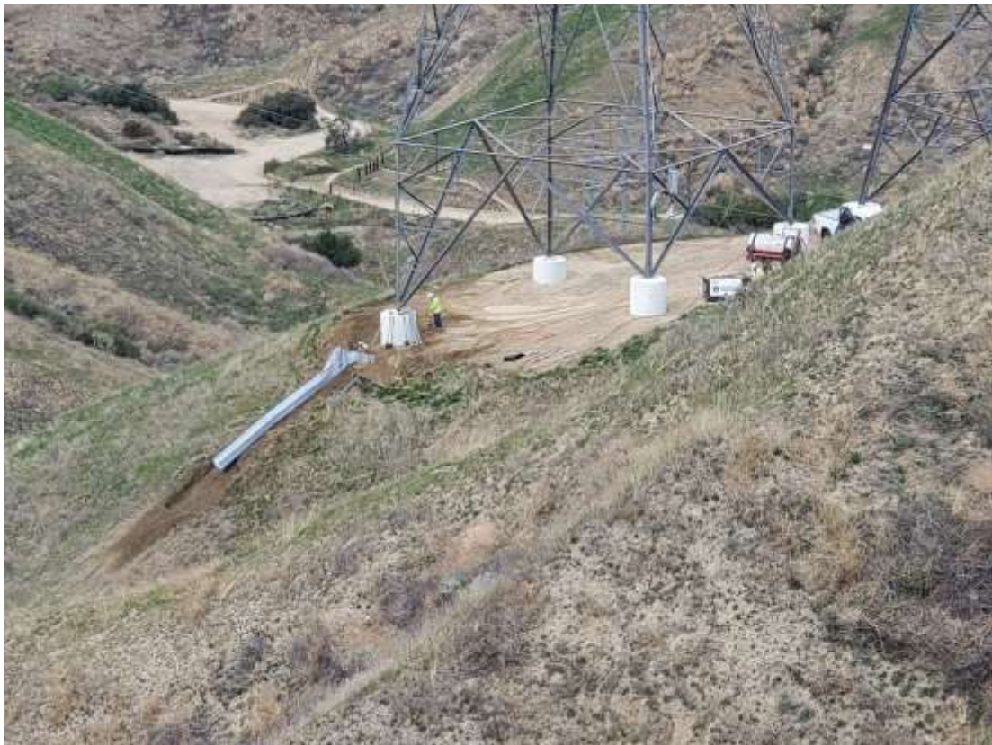
Photo 3 – MAC drain installation at Construction Area 3X65, Segment 3 (March 8, 2021).
