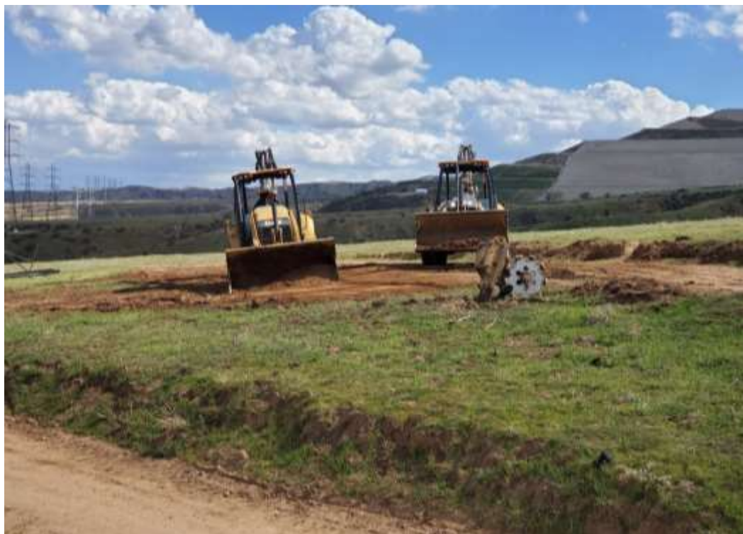
Photo 2 – Foundation wreck-out activities at Construction Area 3X59, Segment 3 (March 9, 2021).
