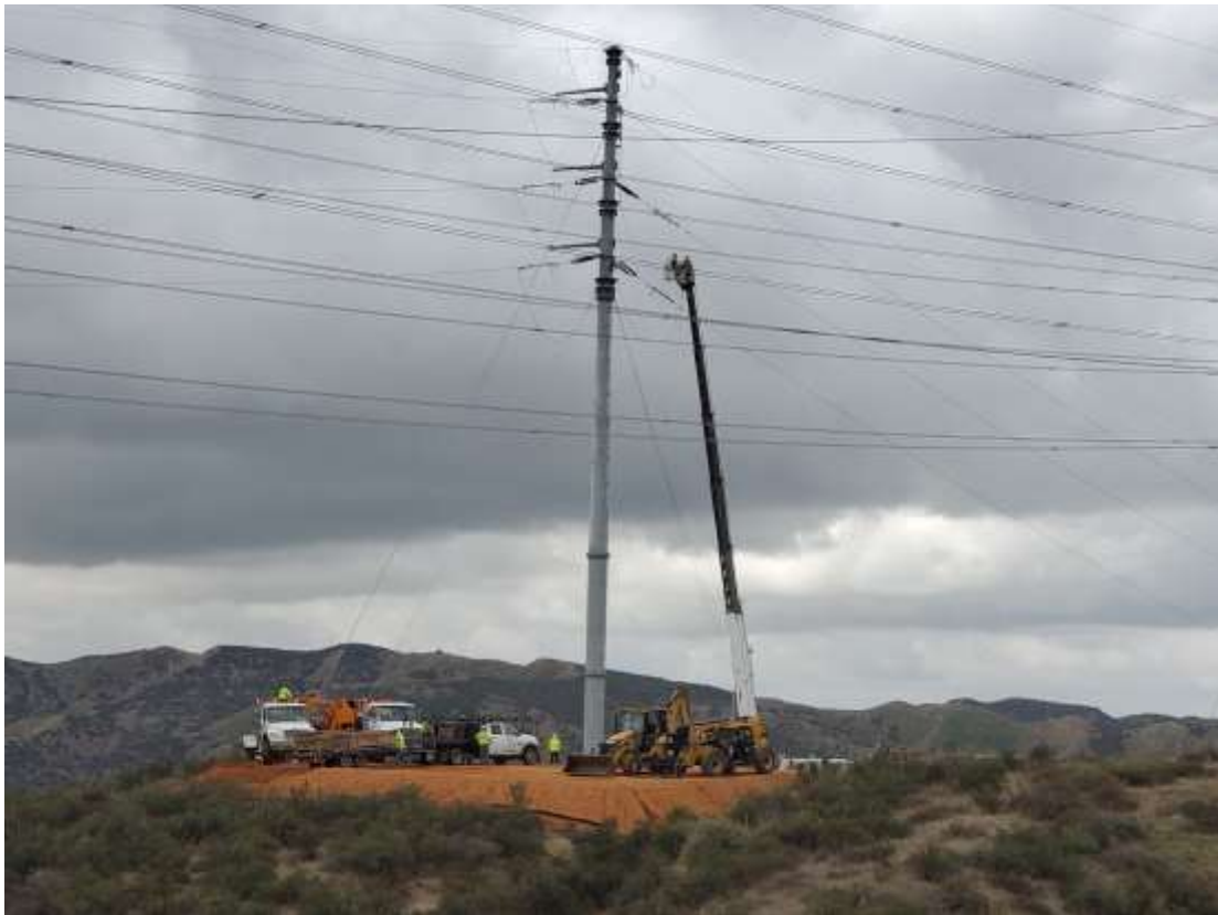
Photo 5 – Wire wreck-out activities at Construction Area 4X56, Segment 4 (March 8, 2021).
