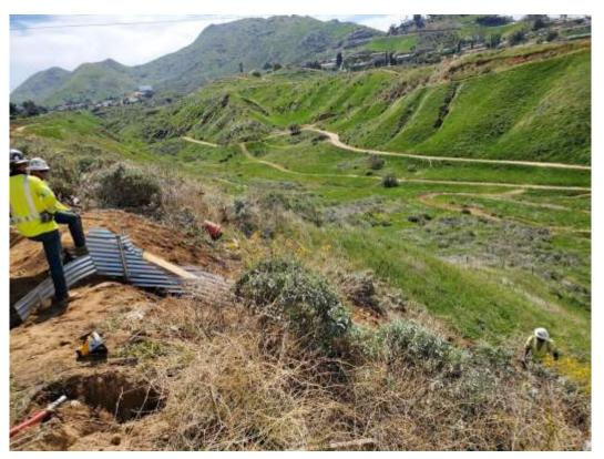
Photo 1 – MAC drain installation at Construction Area 2N25, Segment 2 (March 17, 2021).
