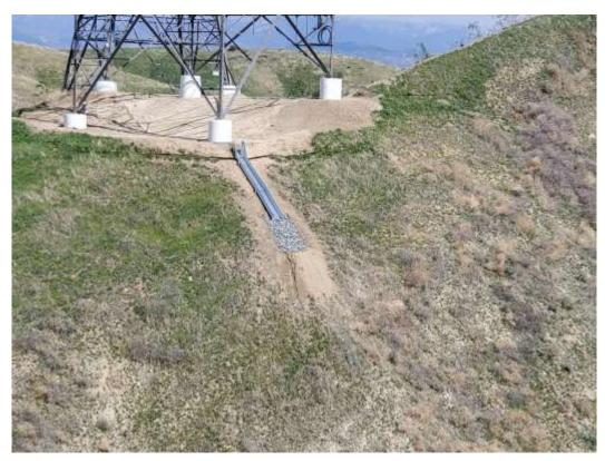
Photo 7 - Erosion downslope of MAC drain at Construction Area 3X65, Segment 3 (March 16, 2021).
