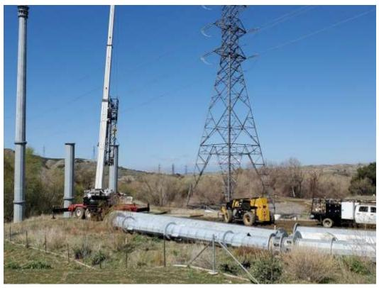
Photo 3 – Shoofly tower wreck-out at Construction Area 4S60, Segment 4 (March 16, 2021).
