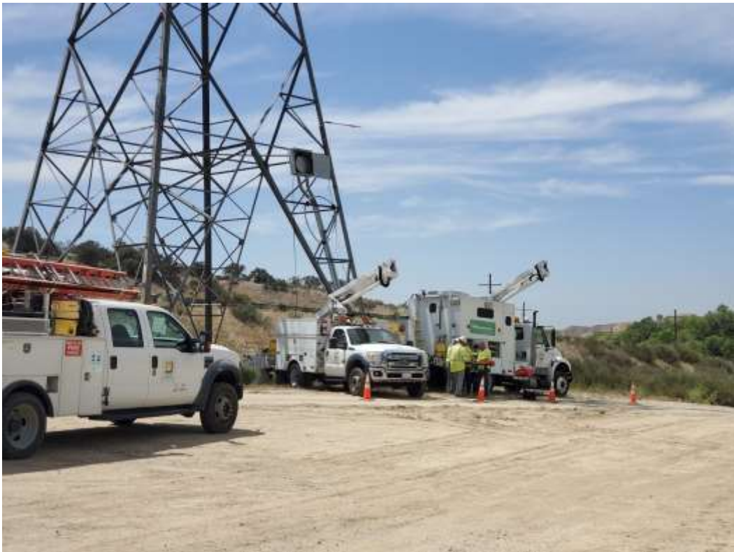
Photo 3 – Fiber optic testing at Construction Area 3N01, Segment 3 (May 5, 2021).
