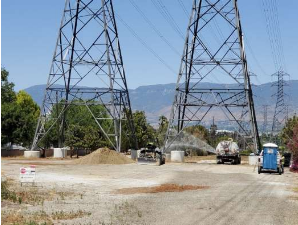
Photo 1 – Site restoration activities at Construction Area 1X08, Segment 1 (May 3, 2021).
