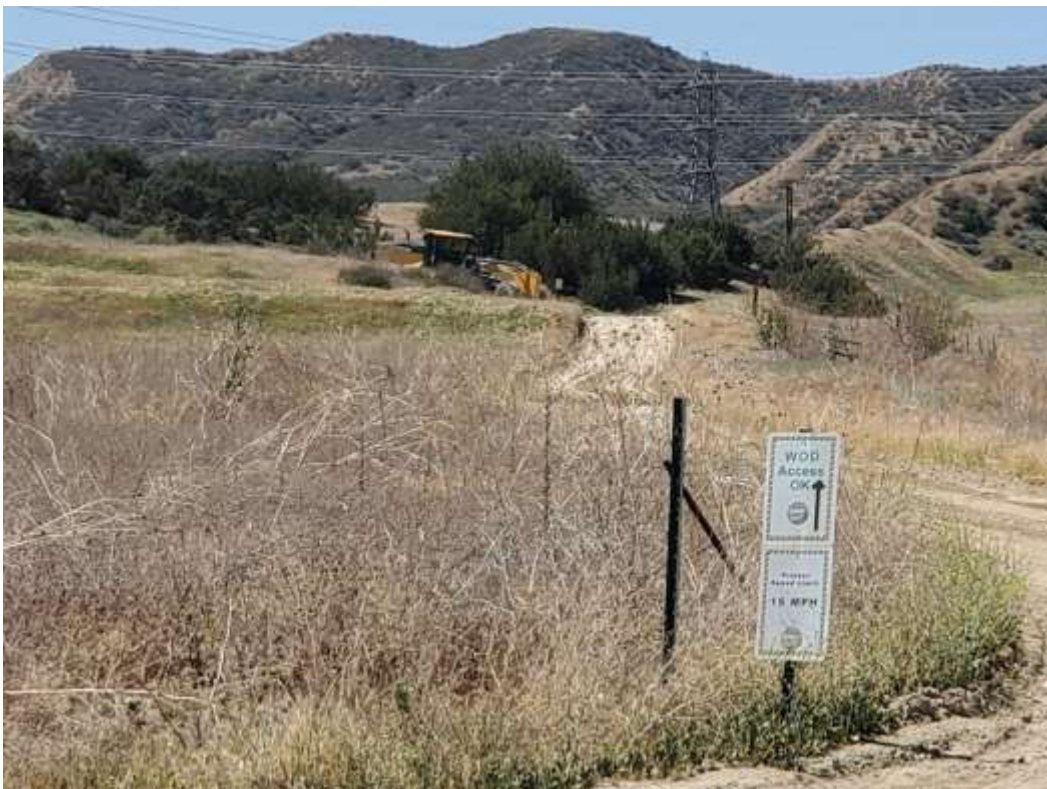
Photo 2 – Maintenance on the access road to Construction Area 3X06, Segment 3 (May 3, 2021).
