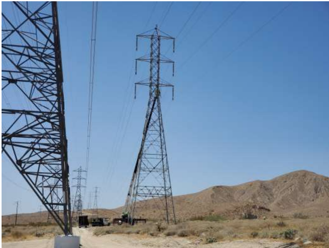
Photo 5 – Wire wreck-out activities at Construction Area 5X04, Segment 5 (May 6, 2021).
