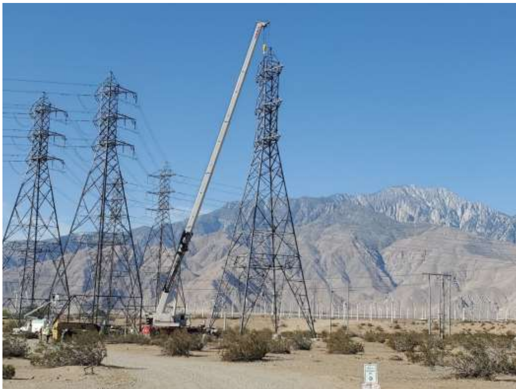
Photo 6 – Tower wreck-out activities at Construction Area 6X09-6X10, Segment 6 (May 5, 2021).
