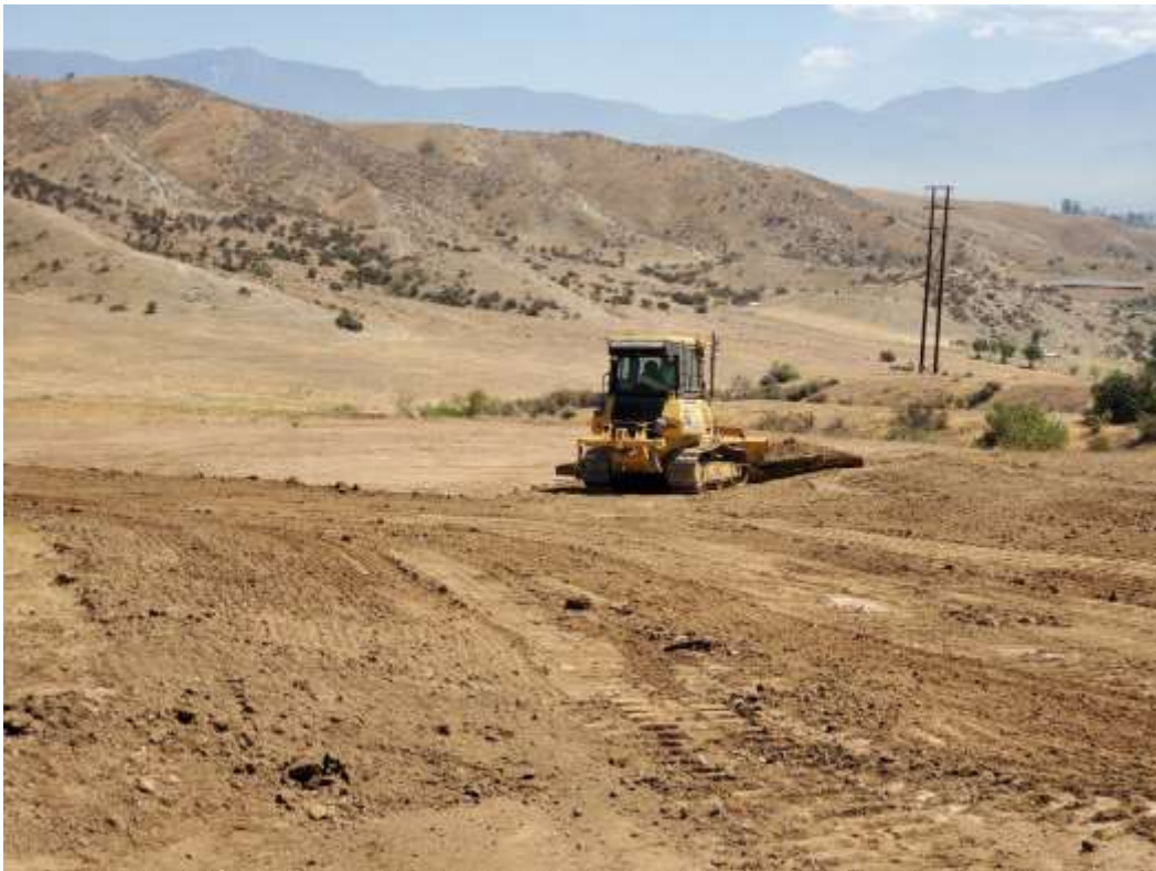
Photo 3 – Site restoration activities at Construction Area PP123229, Segment 3 (June 1, 2021).
