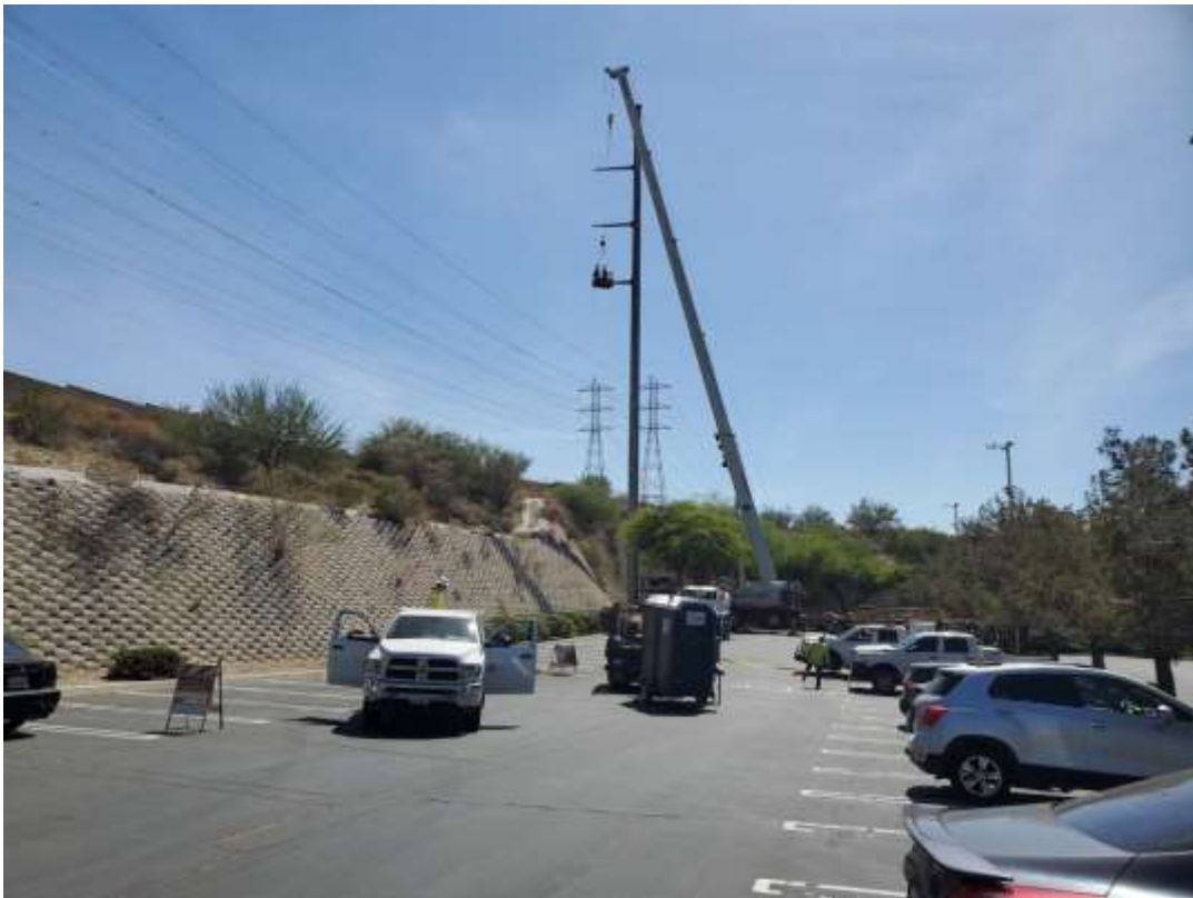
Photo 5 – Tower wreck-out at Construction Area 4175196E, Segment 5 (June 2, 2021).
