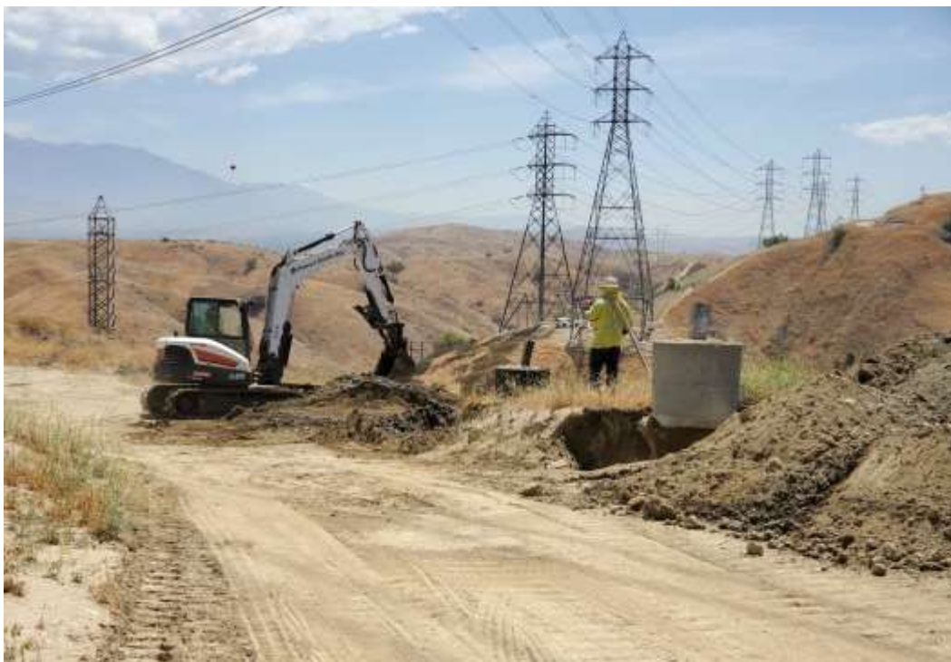
Photo 2 – Foundation wreck-out activities at Construction Areas 2N01 and 2N01-WSS, Segment 2 (June 1, 2021).
