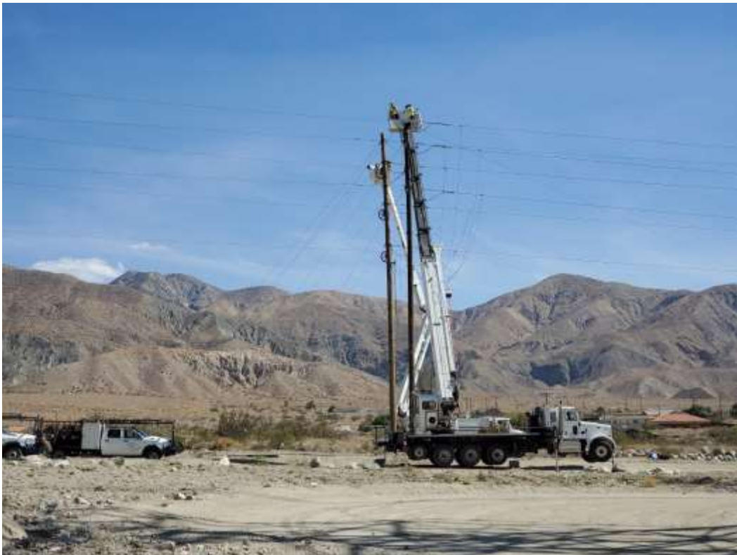
Photo 6 – Wire wreck-out activities at Construction Area 6X42, Segment 6 (June 2, 2021).
