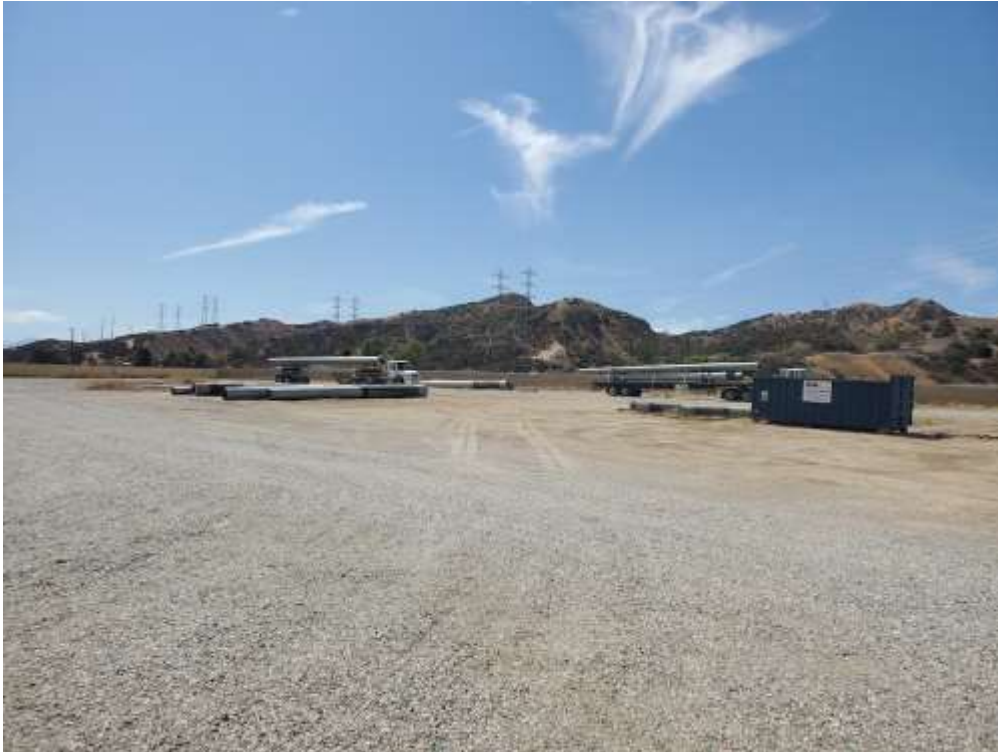
Photo 1 – Material demobilization at the Poultry MY (July 29, 2021).
