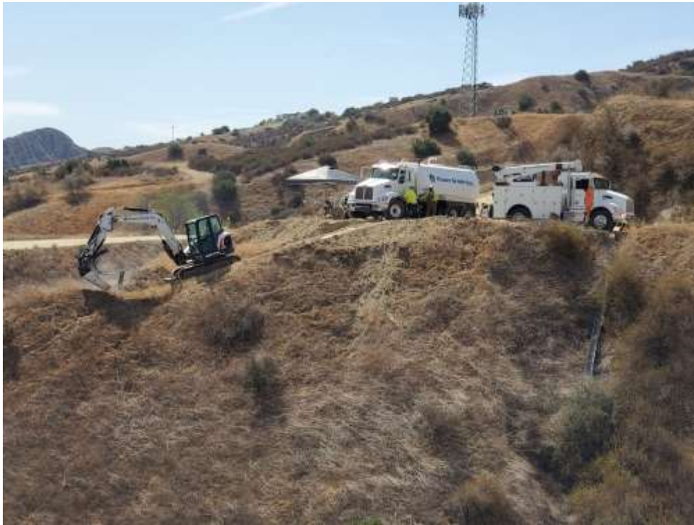
Photo 3 – Foundation wreck-out activities at Construction Area 3X28, Segment 3 (July 29, 2021).
