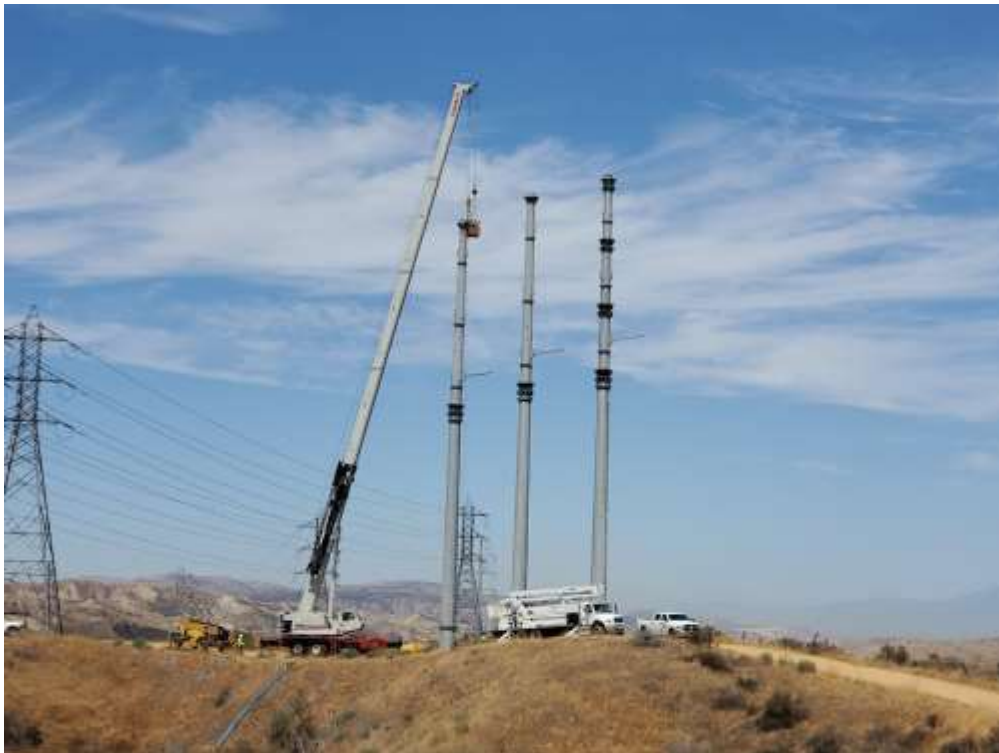
Photo 4 – Tower wreck-out at Construction Area SF411, Segment 4 (July 29, 2021).
