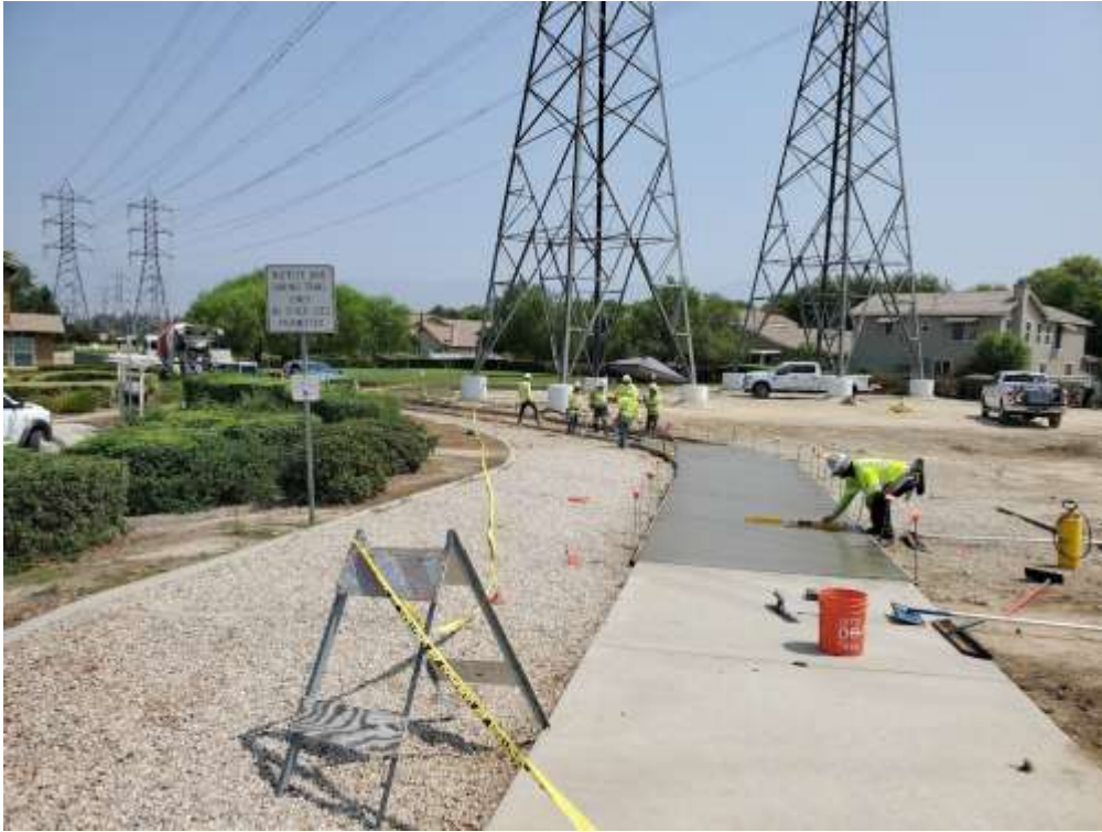
Photo 1 – Concrete replacement activities at Construction Area 1X12, Segment 1 (August 17, 2021).
