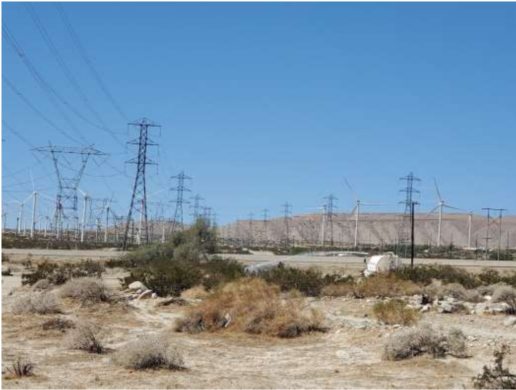
Photo 5 – Hydroseed watering at Construction Area 6N15, Segment 6 (September 15, 2021).
