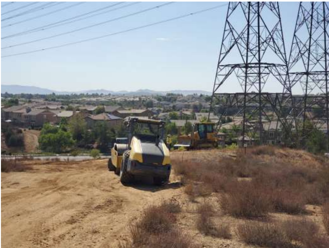
Photo 4 – Site restoration activities at Construction Area 4X53, Segment 4 (September 17, 2021).
