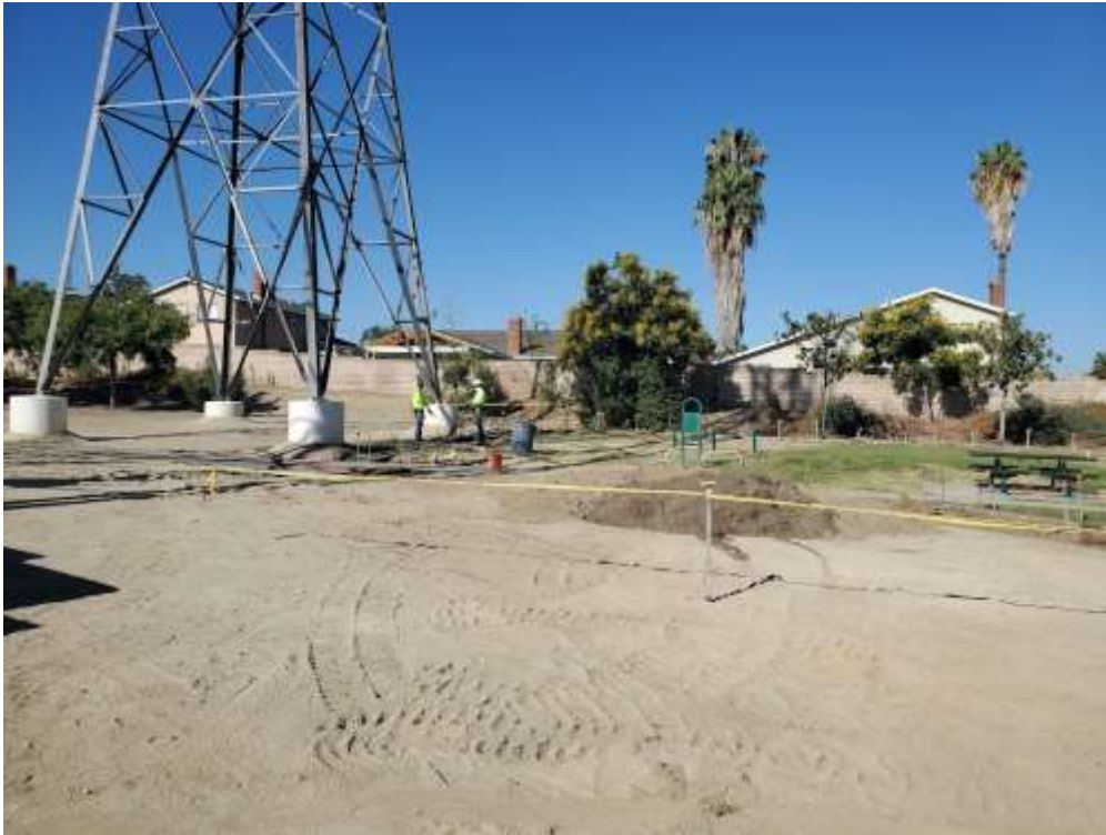
Photo 2 – Concrete repair activities at Construction Area 1X05, Segment 1 (September 15, 2021).
