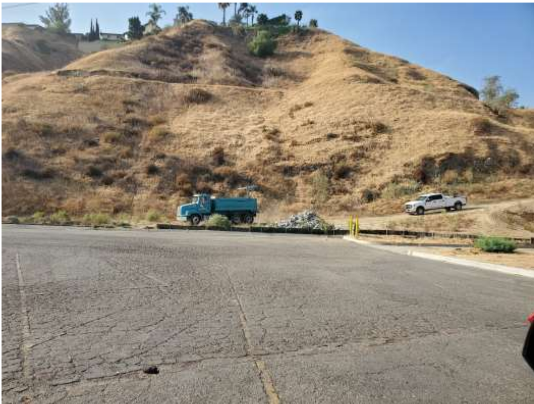
Photo 3 – Rock delivery at Construction Area 2N32, Segment 2 (September 17, 2021).
