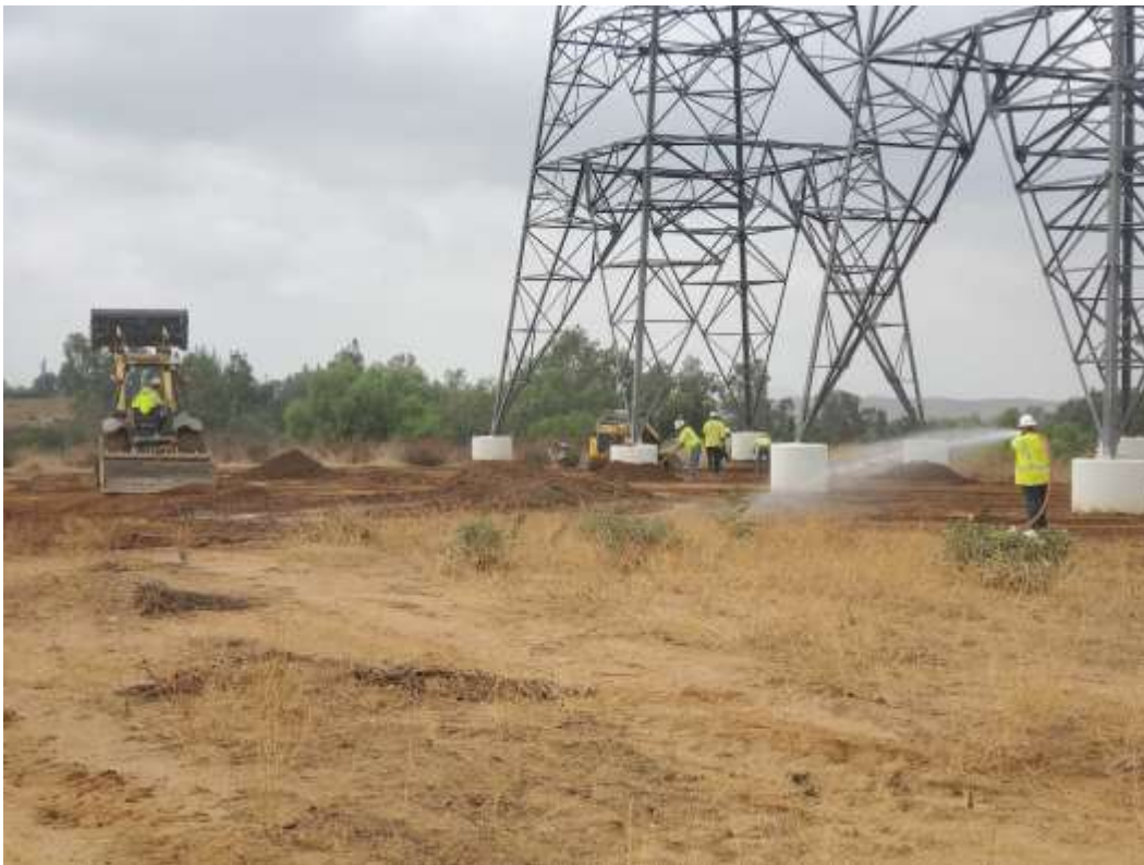
Photo 3 – Site restoration at Construction Area 4X41, Segment 4 (September 28, 2021).
