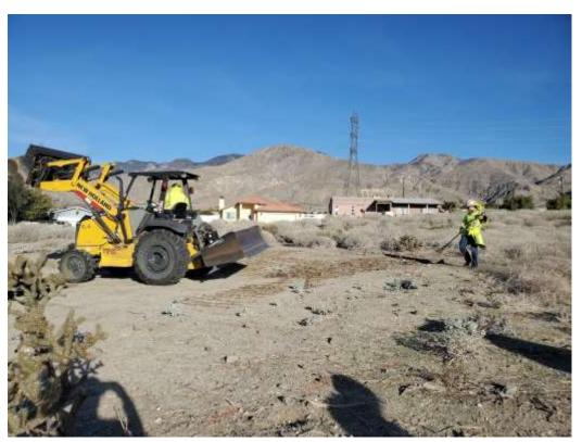
Photo 4 – Site decompaction and hydroseed preparation at Construction Area 6S40, Segment 6 (January 4, 2022).
