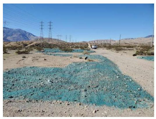
Photo 5 – Hydroseed application at Construction Area 6X11, Segment 6 (January 3, 2022).
