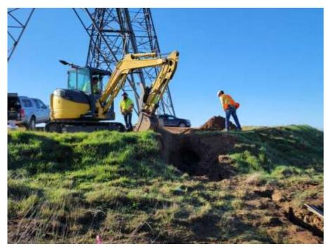
Photo 5 – Exploratory potholing at Construction Area 4X34, Segment 4 (February 16, 2022) (Photo courtesy of SCE).
