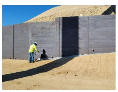
Photo 6 – Patina application at Construction Area 6N31, Segment 6 (February 2, 2022) (Photo courtesy of SCE).
