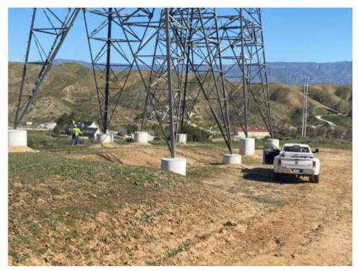
Photo 1 – BMP removal and site clean-up at Construction Area 3X57, Segment 3 (March 9, 2022) (Photo courtesy of SCE).
