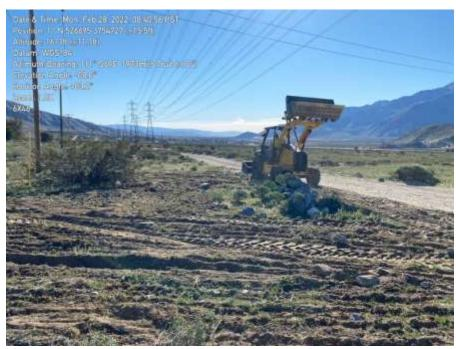
Photo 3 – Decompaction at Construction Area 6X46, Segment 6 (February 28, 2022) (Photo courtesy of SCE).
