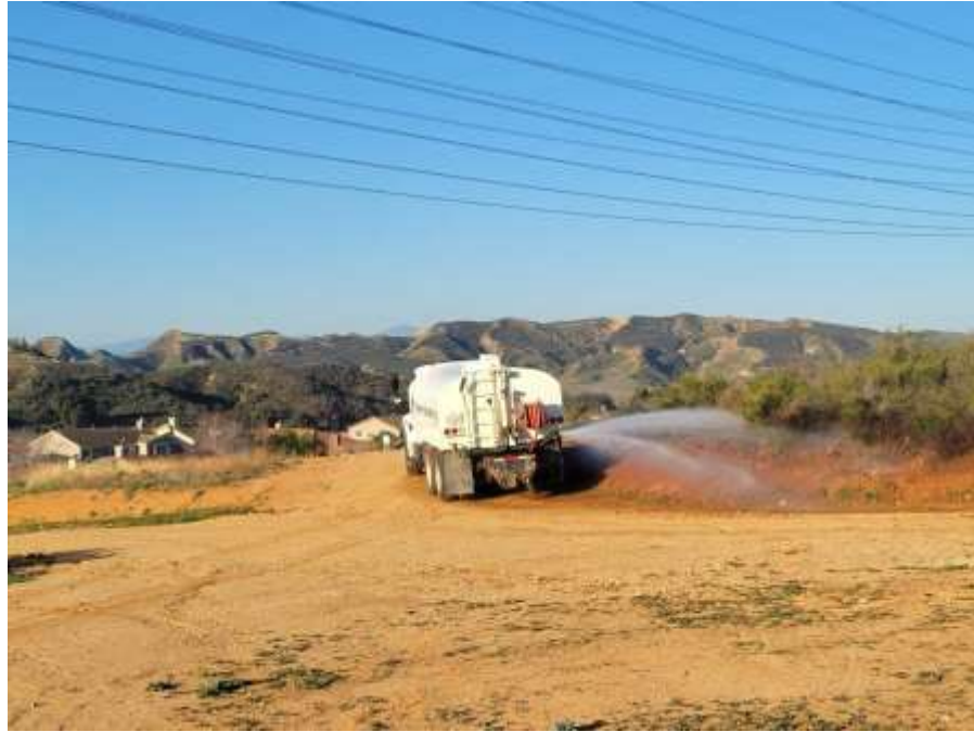
Photo 3 – Hydroseed watering at Construction Area 4X52, Segment 4 (March 14, 2022) (Photo courtesy of SCE).
