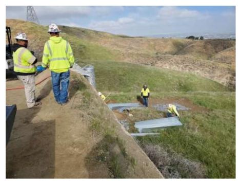
Photo 1 – Erosion repair and MAC drain installation at Construction Area 2N11, Segment 2 (March 30, 2022).
