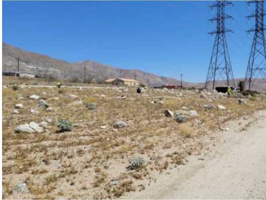
Photo 3 – Hand weeding at Construction Area 5X01, Segment 4 (April 13, 2022) (Photo courtesy of SCE).
