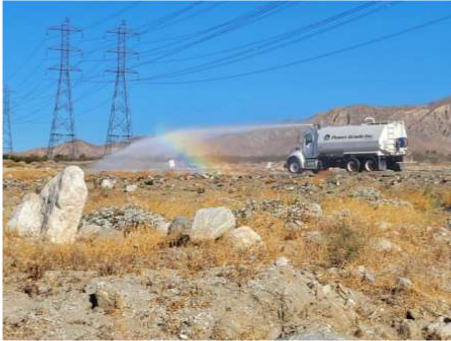
Photo 5 – Hydroseed watering at Construction Area 6X42, Segment 6 (June 7, 2022) (Photo courtesy of SCE).
