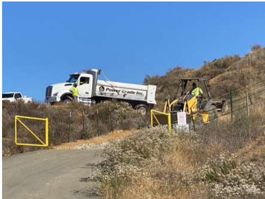
Photo 4 – Stabilized entrance removal at Palmer Avenue, Segment 4 (June 20, 2022) (Photo courtesy of SCE).
