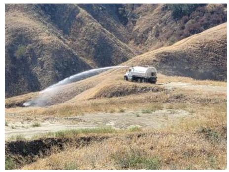
Photo 3 – Hydroseed watering at Construction Area 2N01, Segment 2 (June 28, 2022) (Photo courtesy of SCE).
