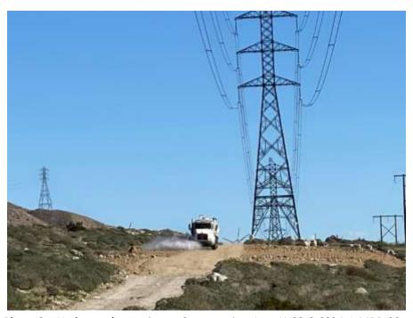
Photo 2 – Hydroseed watering at Construction Area WSS-6-6S34-1-MPR-29, Segment 6 (December 12, 2022) (Photo courtesy of SCE).
