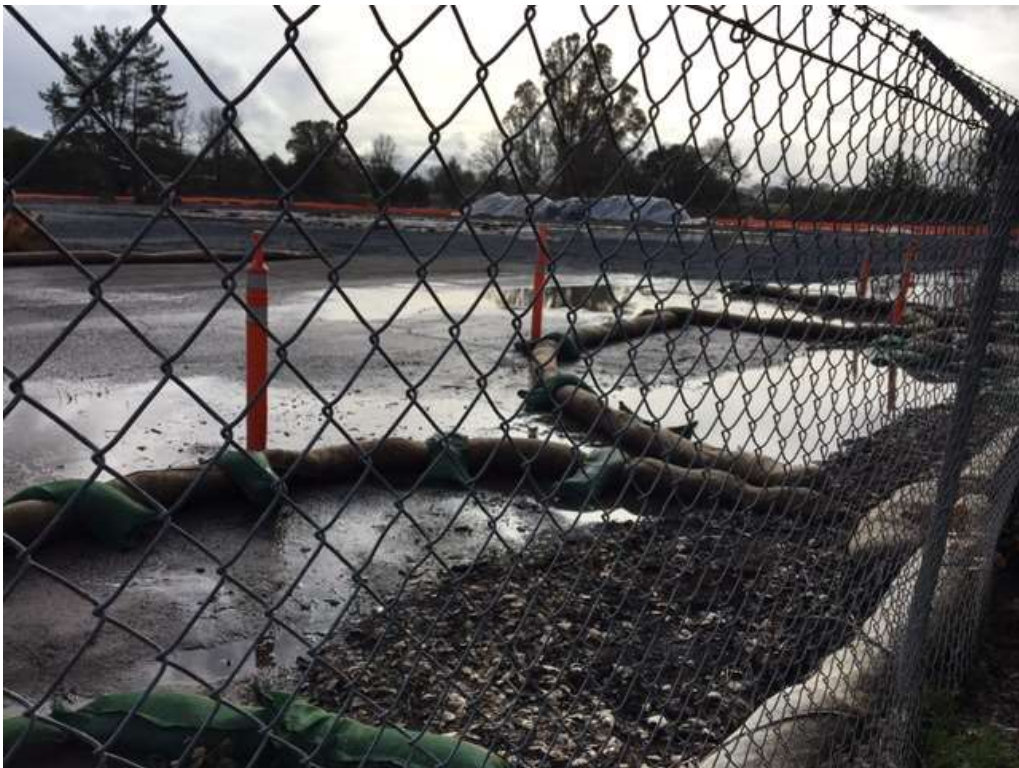
Figure 4 – Drainage inlets on the northern side of the substation site, January 11, 2017.
