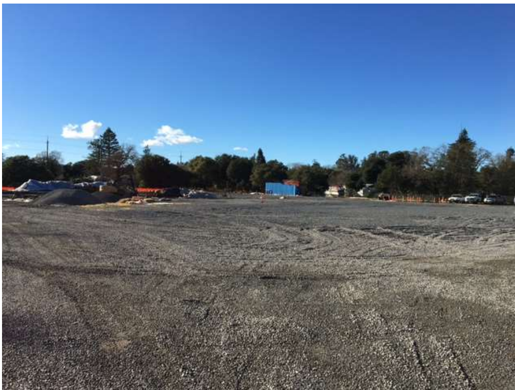
Figure 1 – Base rock compacted at substation site – view west-northwest, January 5, 2017.
