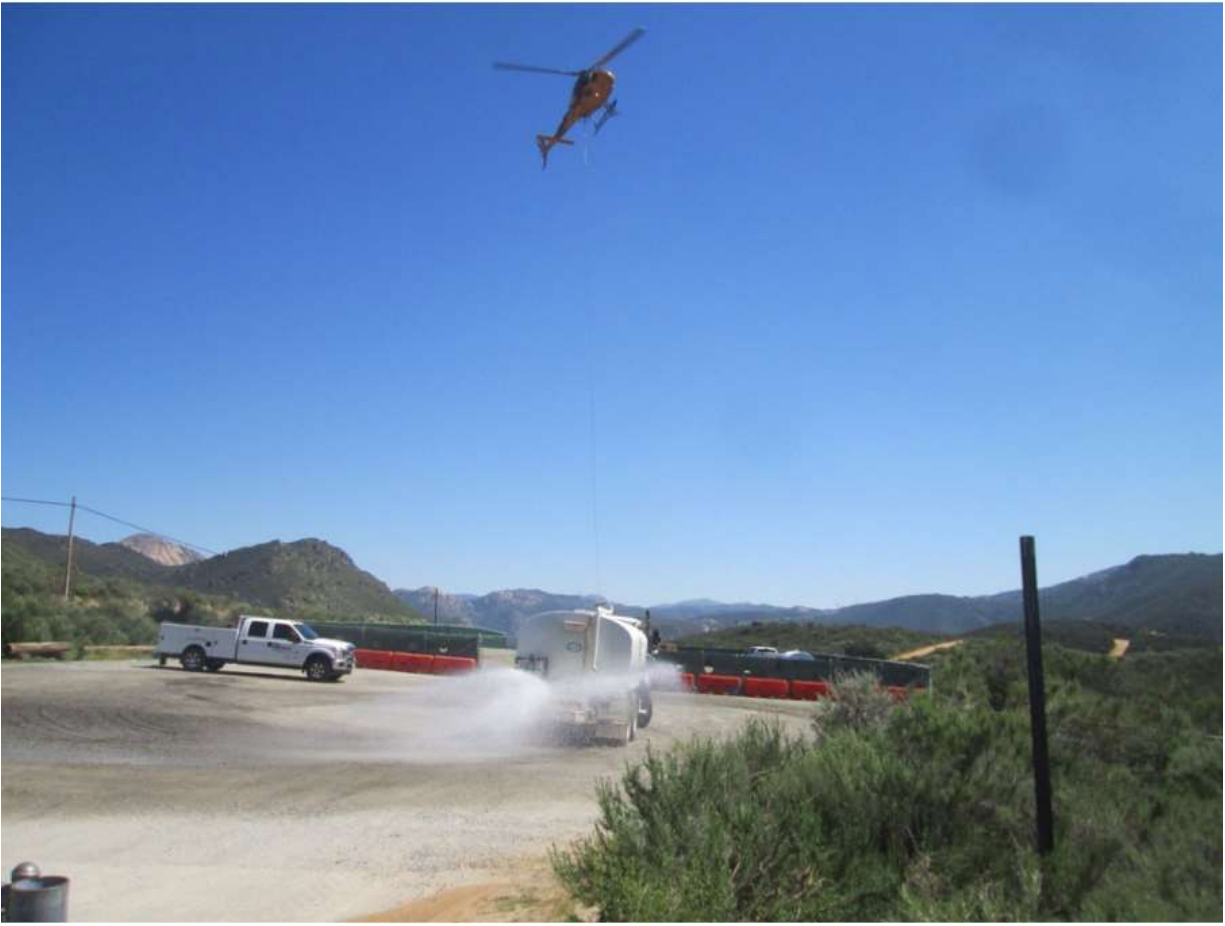
Photo 2: During helicopter staging and external load operations at Sweetwater Staging Area, a water truck was utilized to minimize dust emissions, and a ground crew member was present to ensure safety in accordance with MM-PHS-5
