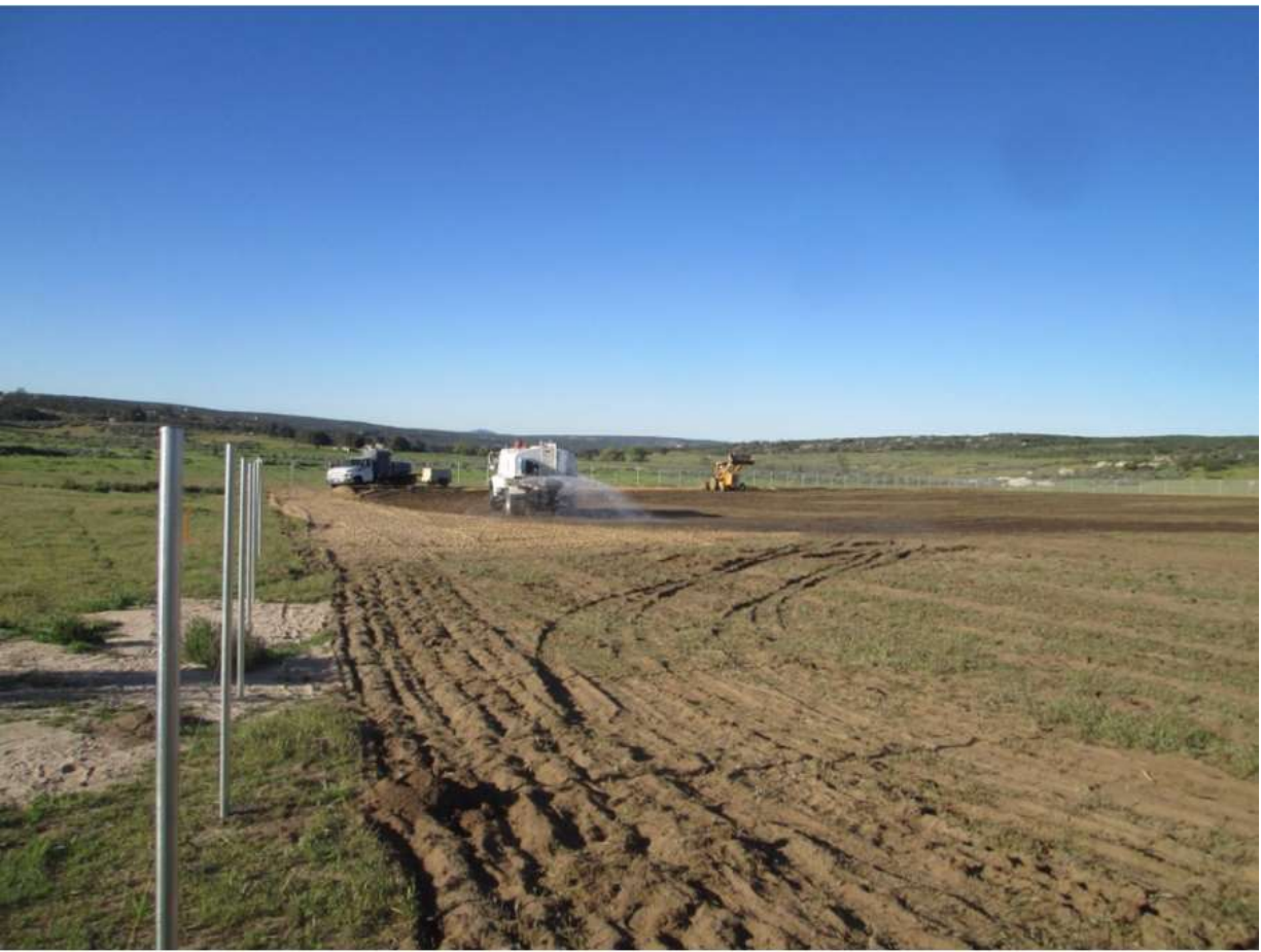
Photo 1: In accordance with APM-AIR-02, a water truck was observed being utilized to apply water in Live Oak Springs Staging Yard to prevent dust emissions.
