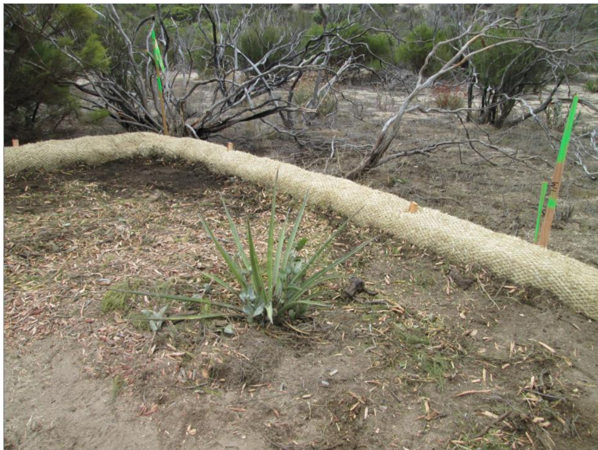
Photo 6: Crews were observed avoiding plants designated for salvage as described in the HRP and SSPSRP (MM BIO- 4, MM BIO-15). Salvaged plants were observed being transported to an off-site nursery until the restoration phase for the segment. Fiber rolls were placed around work sites as approved in the SWPPP (APM HYD-05, MM BIO-7, MM HYD-1).
