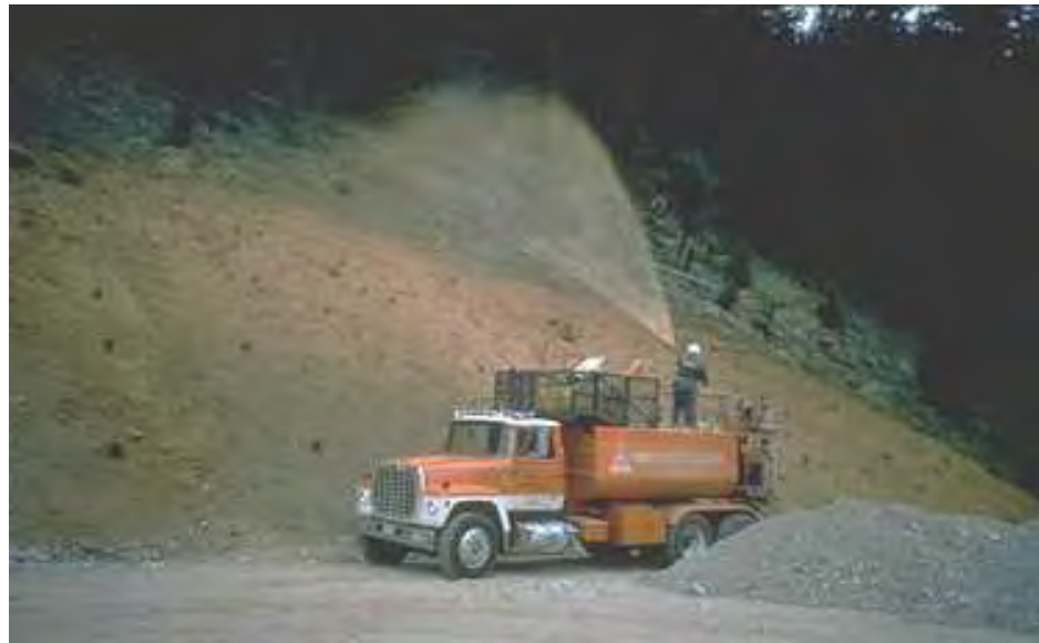
Applying hydraulic mulch.
