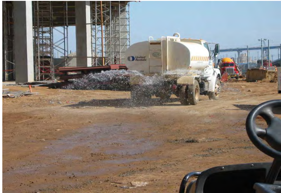
Water being applied for dust control.
