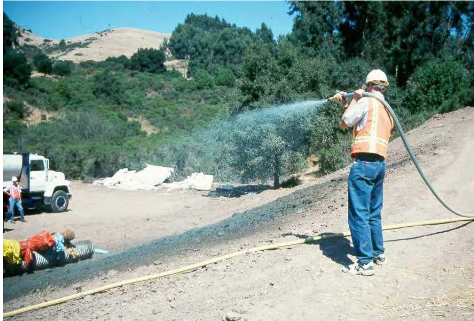
Applying hydroseed.
