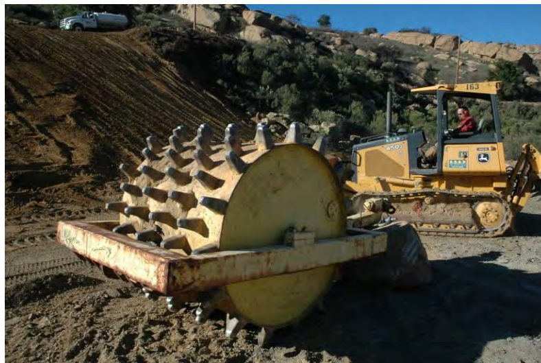
Sheepsfoot used for soil preparation
