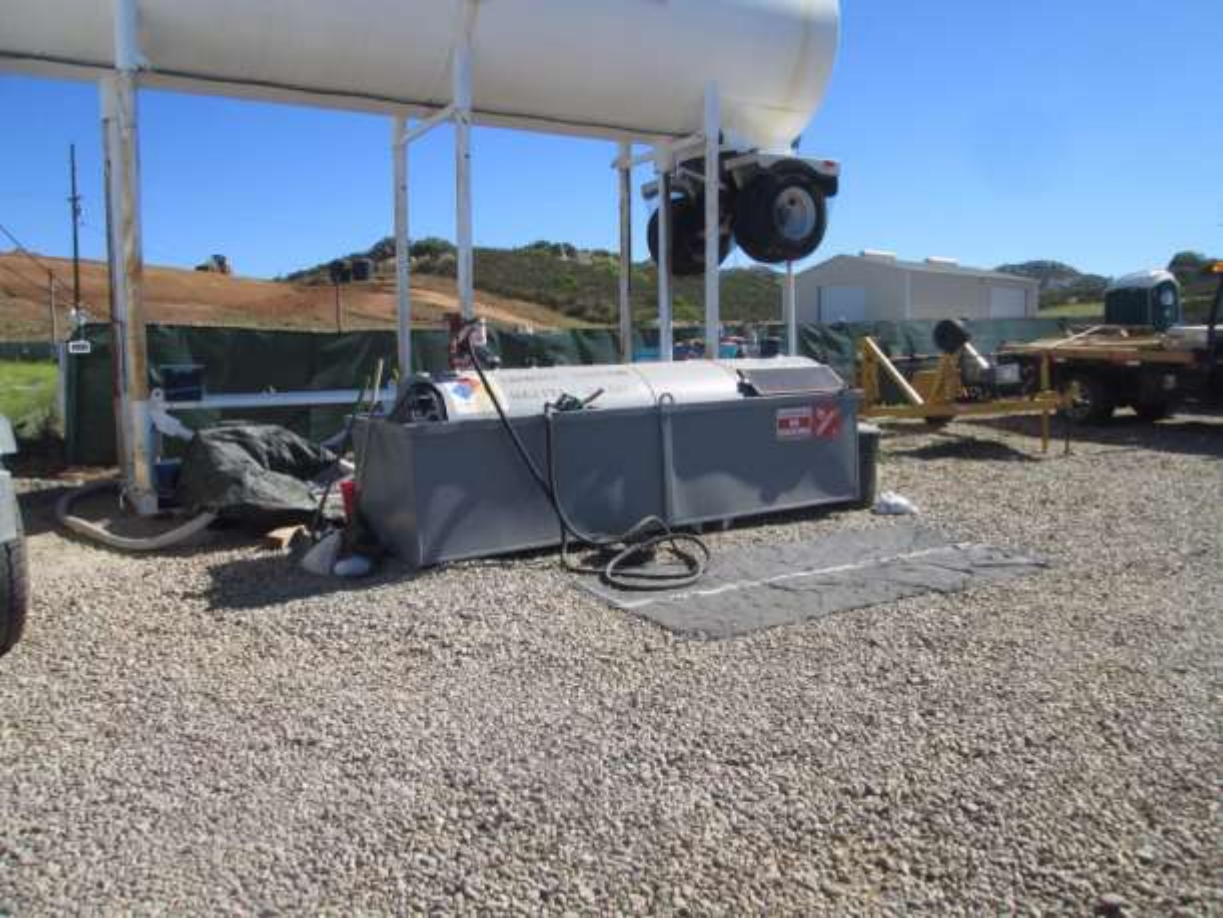
Photo 4: Fuel is stored in secondary containment at Japatul Spur Staging Area in accordance with MM PHS-2 and the SWPPP.
