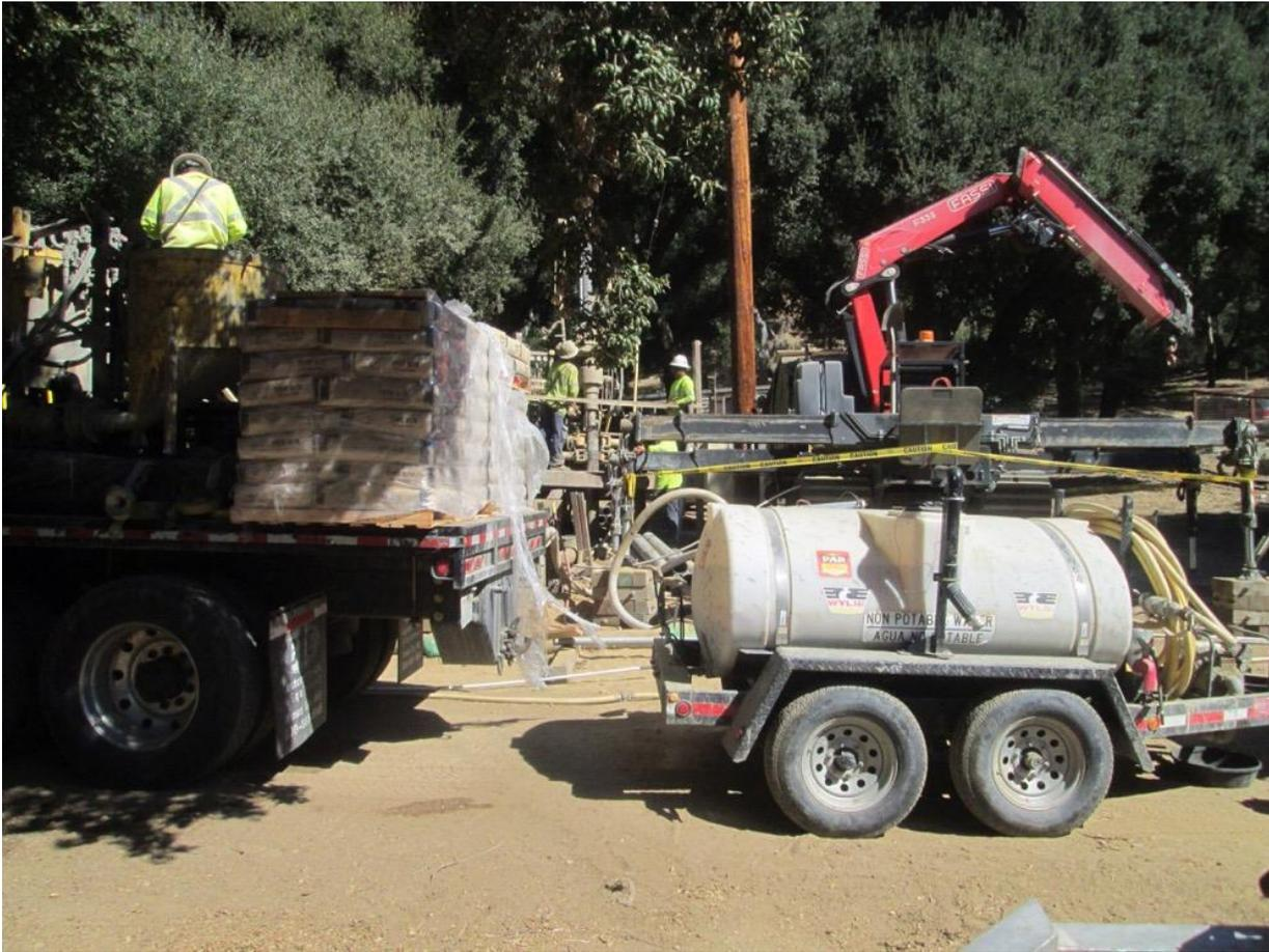
**Photo 4:** During grouting activities at Z118122, a water buffalo was used to capture and contain concrete wash water in accordance with APM-HYD-01 (TL 682).
