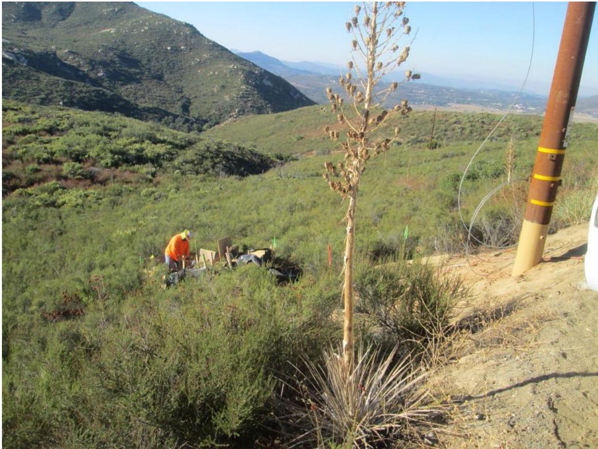
**Photo 1:** Anchor hole digging was observed at P172687. Work and access occurred within the delineated limits of disturbance in accordance with MM BIO-1 (C 78).
