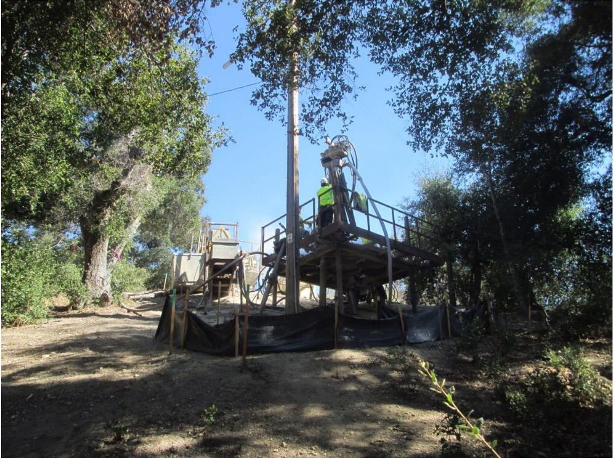
**Photo 3:** A silt fence was observed around the downslope side of the micropile drilling workspace at Z118123 in accordance with the SWPPP (TL 682).
